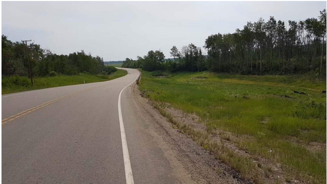
Photo 1 – Looking east over repaired highway and toe berm.
