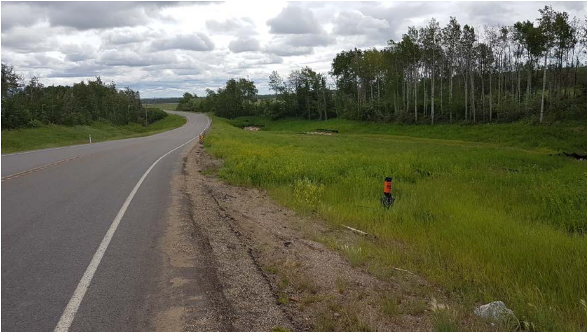
Photo 1 – Looking east over repaired highway and toe berm.
