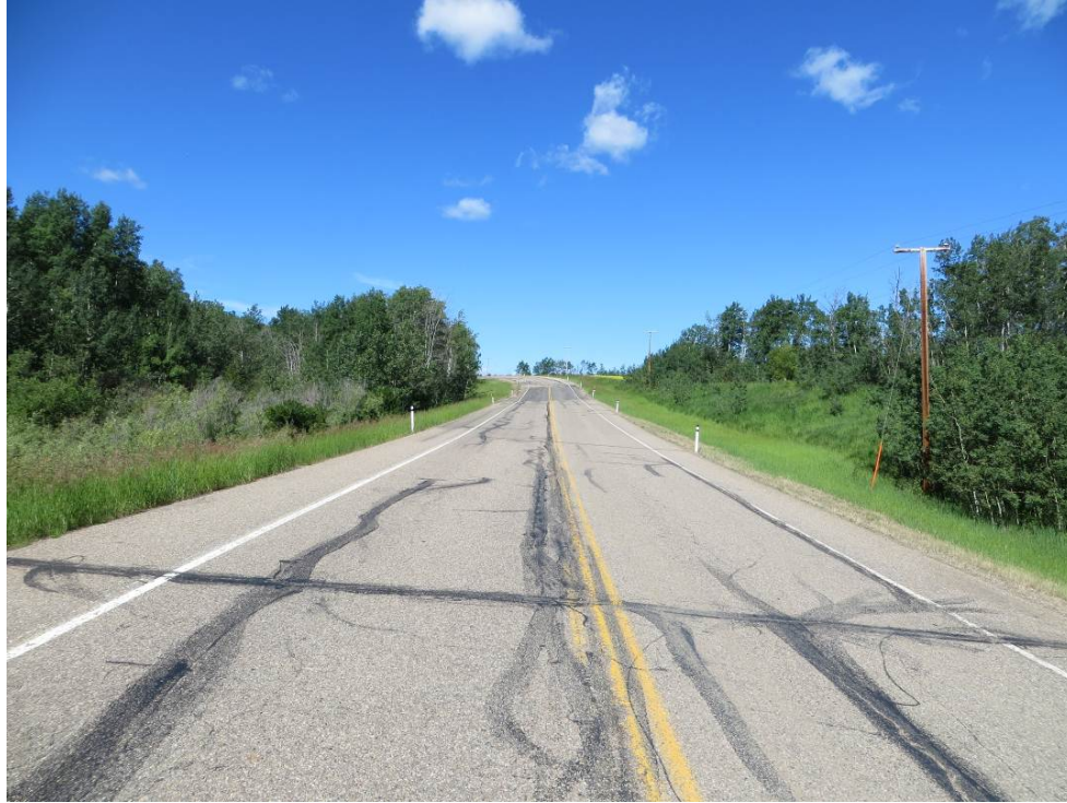
Photo 3 - View of Highway 690 showing the 2011 ACP patch, looking west.
