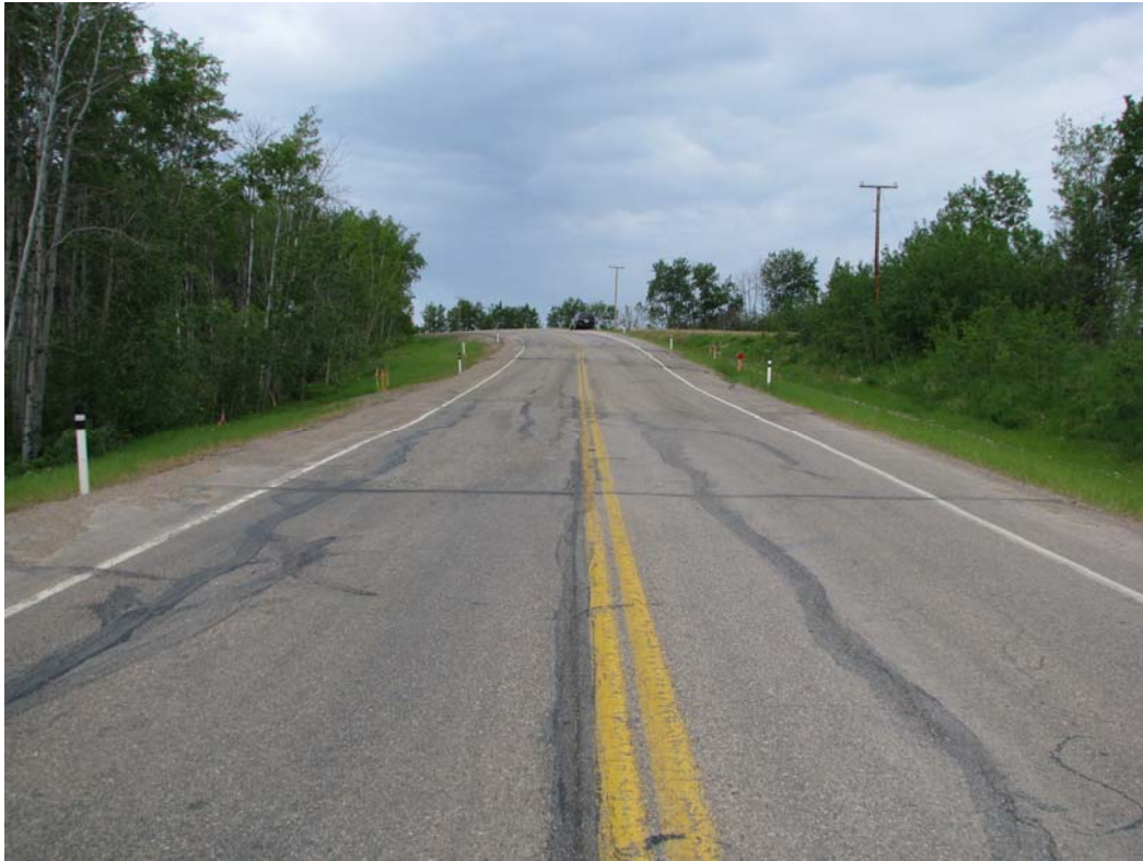
Photo 3 - View of Highway 690 showing the 2008 ACP patch, looking west.
