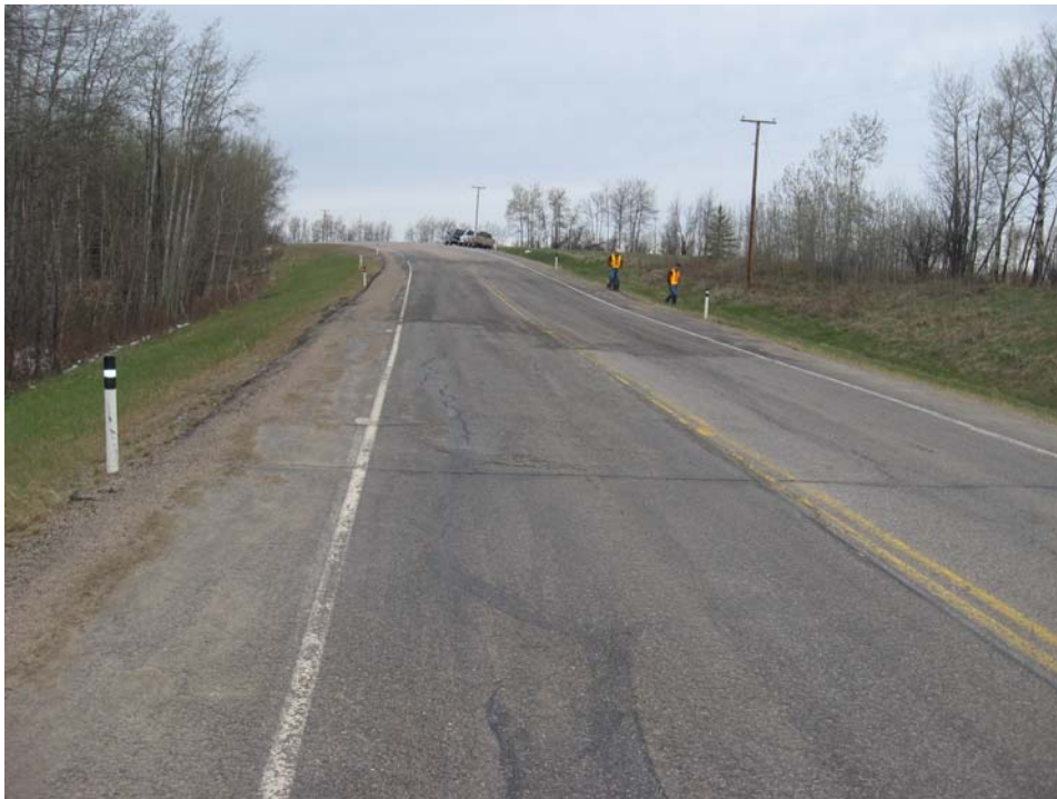
Photo 4 - View of Highway 690 showing the 2008 ACP patch, looking west.
