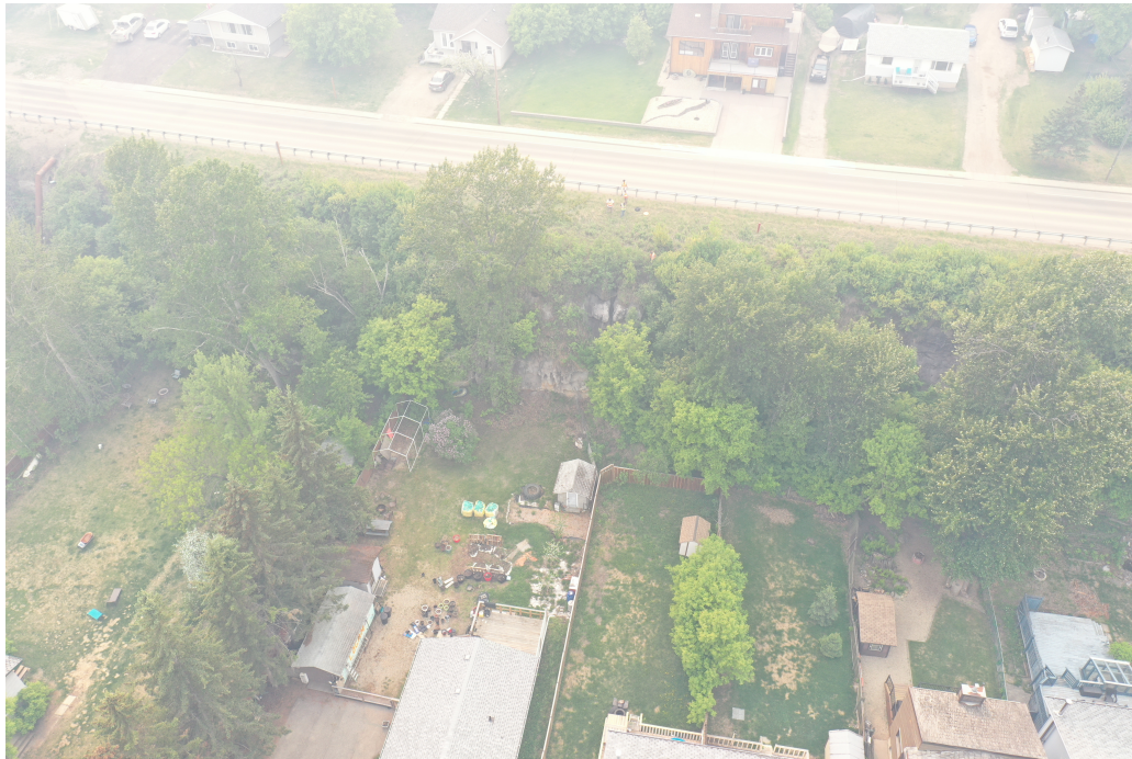
Photo 54-1. Drone photo looking west at location where slope sloughed/eroded in past.
