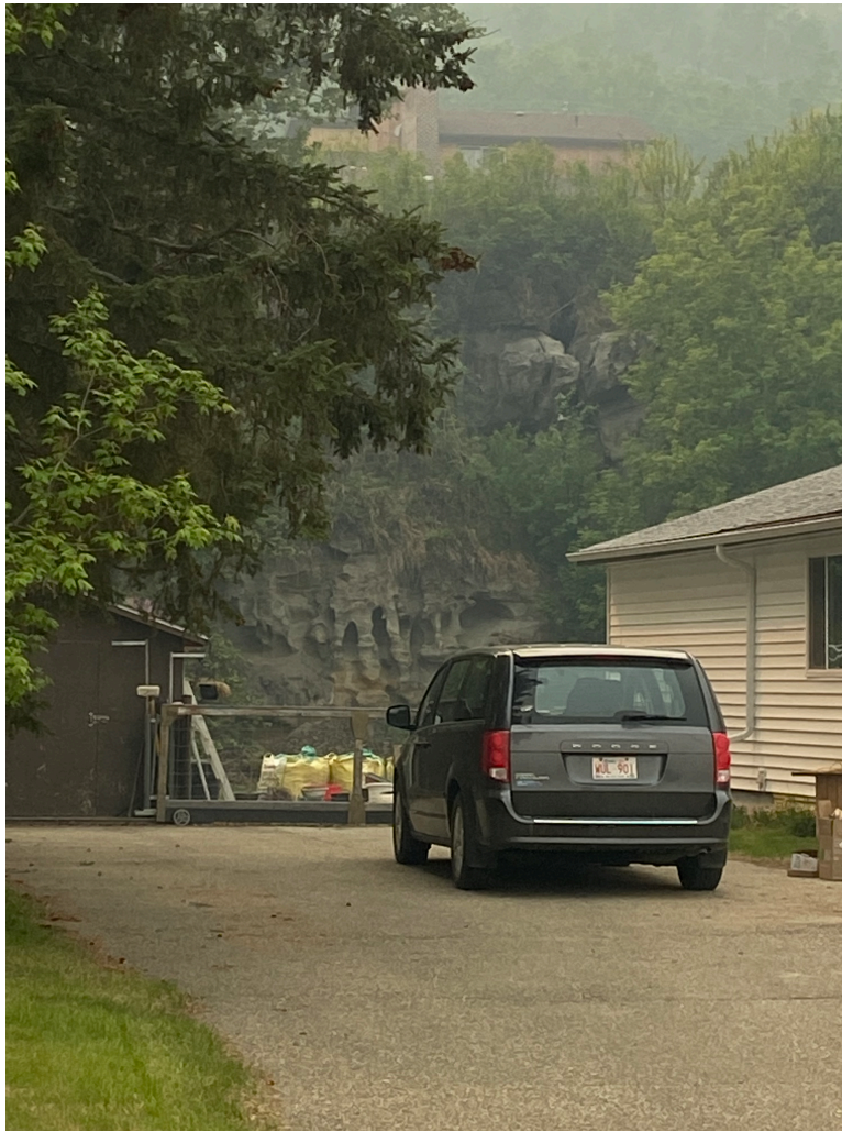
Photo 54-3. Looking west toward lower part of eroded sandstone slope.
