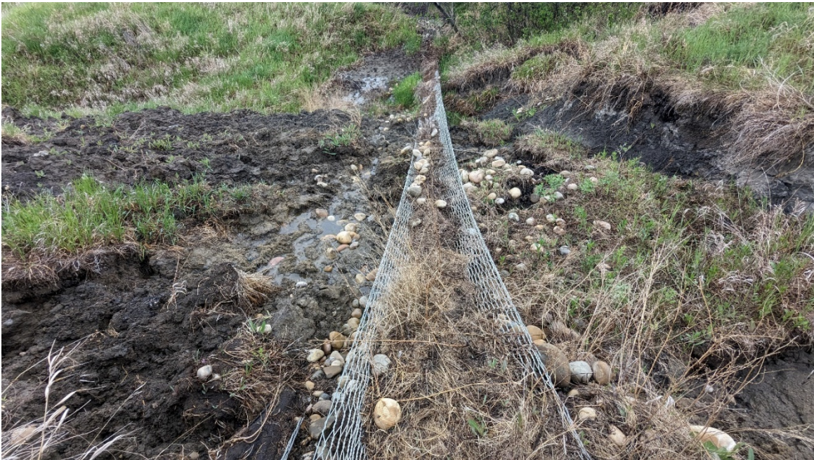
Photo 6: Stretching gabion mattress along the west flank of the landslide.
