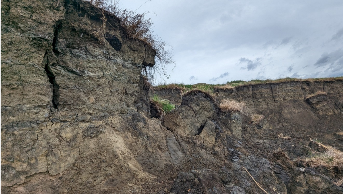
Photo 9: Toppling blocks at the face of the main headscarp.
