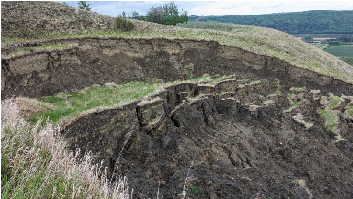
Photo 11: Looking southeast at the east flank of the main landslide.
