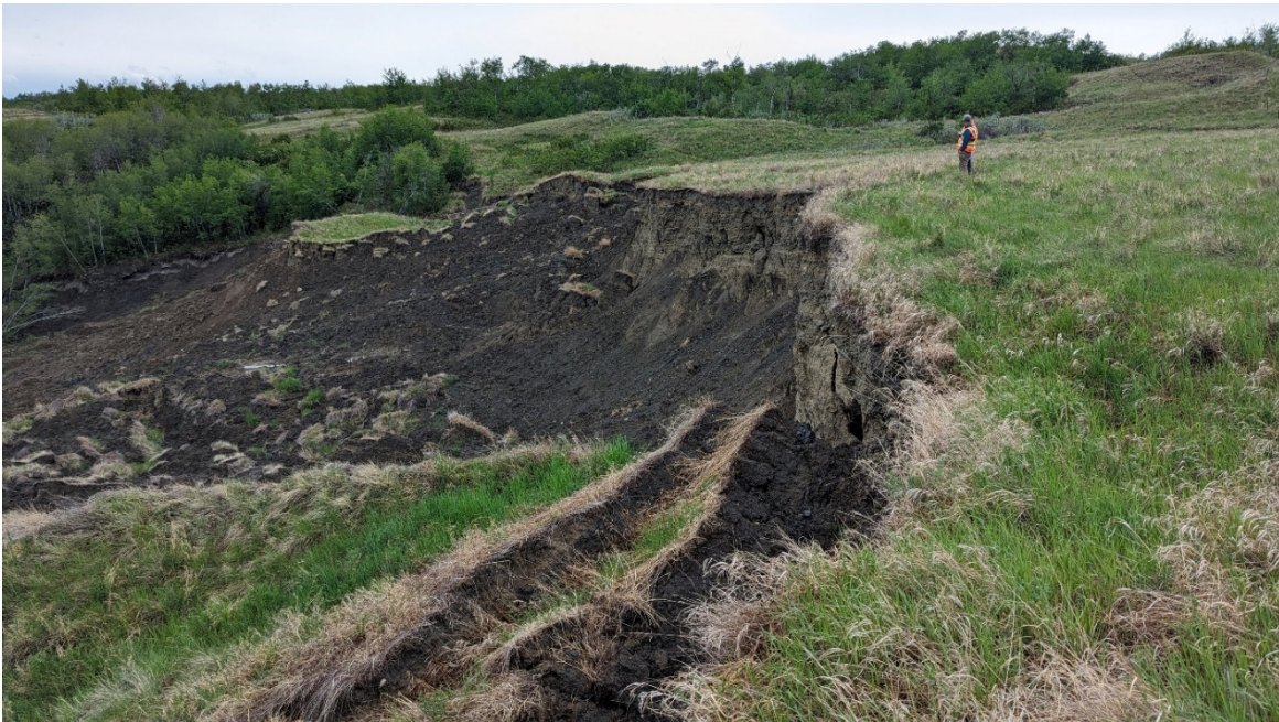
Photo 12: Looking west at the main landslide headscarp.
