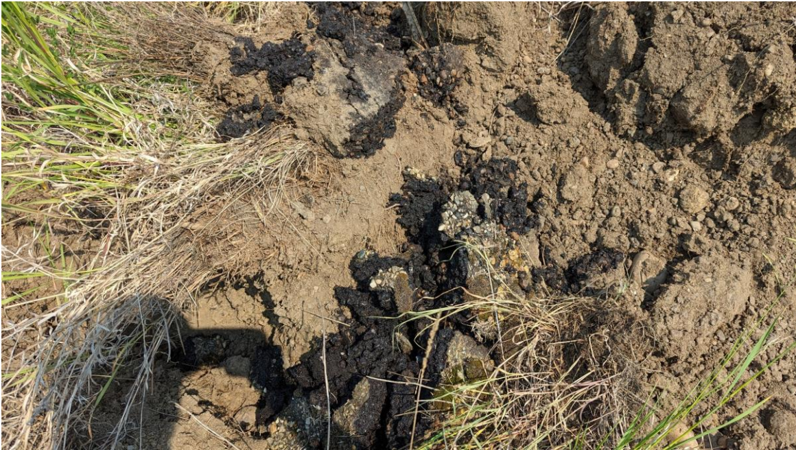
Photo 15A: Pieces of asphalt exposed in the slide debris.
