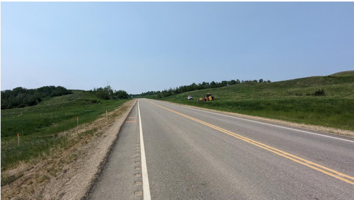
Photo 26: Looking west along as-yet undisturbed highway surface. The proposed temporary detour will be constructed to the right (north) on the flatter terrain. A probable long-term realignment would cut into the hillside further north.
