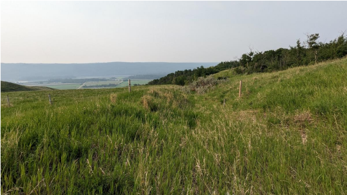
Photo 1: Looking south along grassed drainage channel below centerline culvert.
