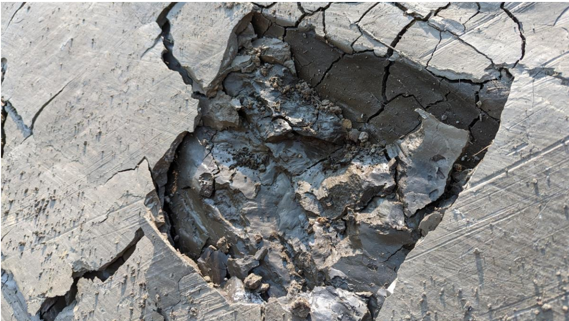
Photo 24B: Moisture on slickensides below the desiccated crust.
