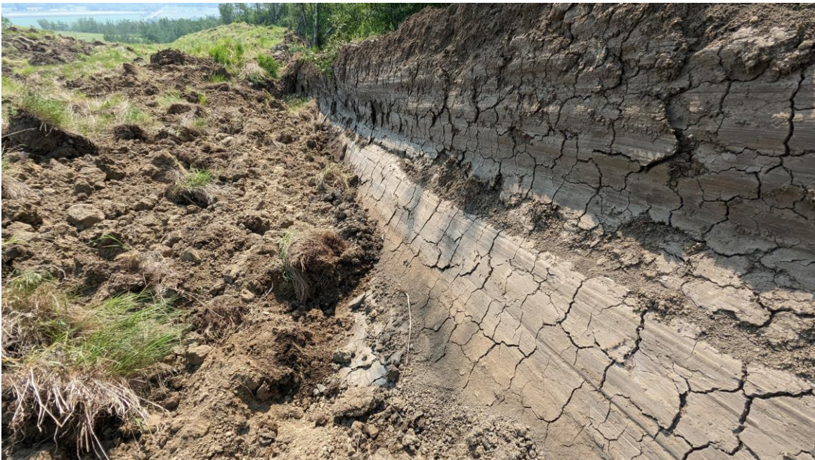
Photo 23: Exposed western flank of the desiccated slip surface.
