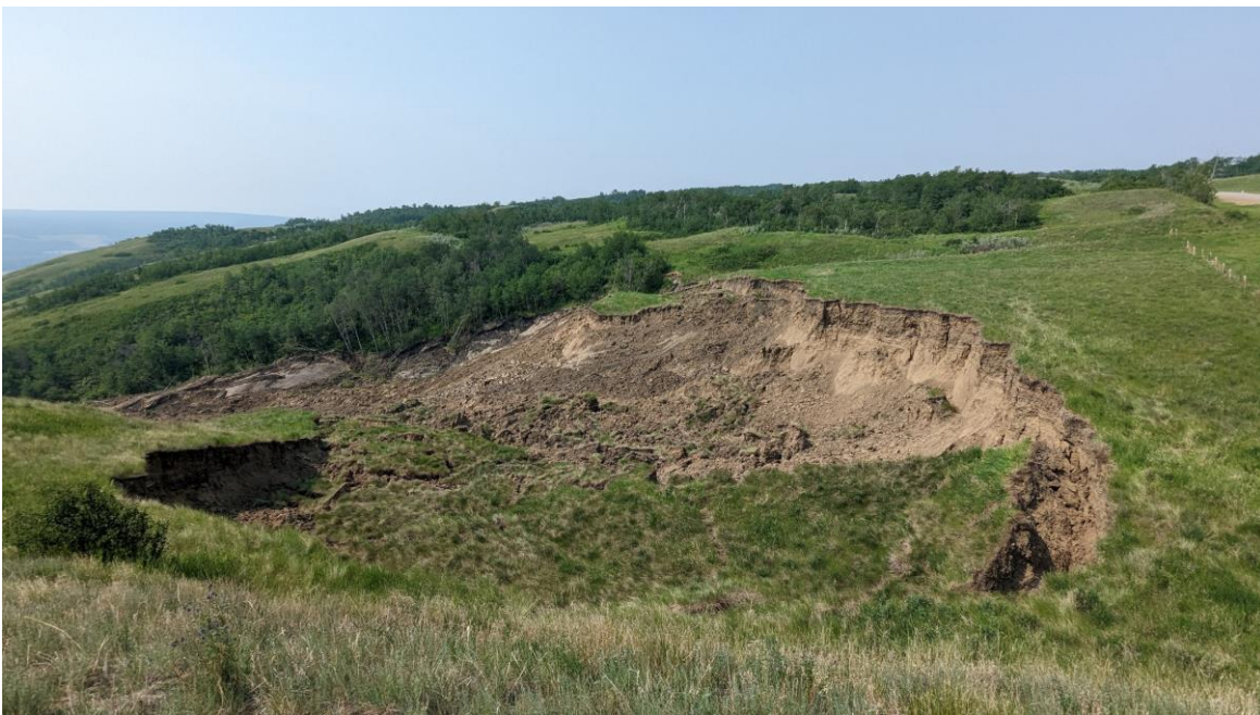
Photo 10: Looking down southwest at the main headscarp.
