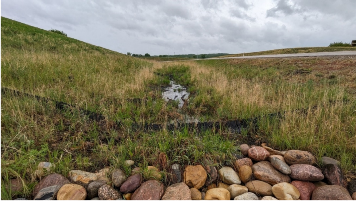
Photo 3 – Looking northwest at repaired ditched along Hwy 2 off-ramp.
