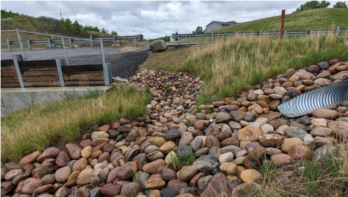
Photo 5: Looking south at NW end of wall just below S111-01 which continues to move even after construction is completed.
