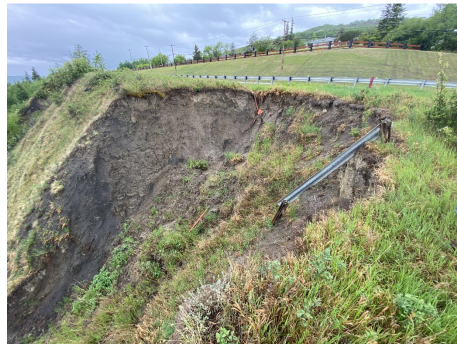
Photo 1. Looking southwest from the north flank of Slide 1. Some fresh soil was visible in the upper scarp/south flank and there was 0.2 m retrogression since 2023. Minimum offset from the main scarp to the guardrail was measured at 3.2 m. Gas marker post has now fallen into the slide area.
