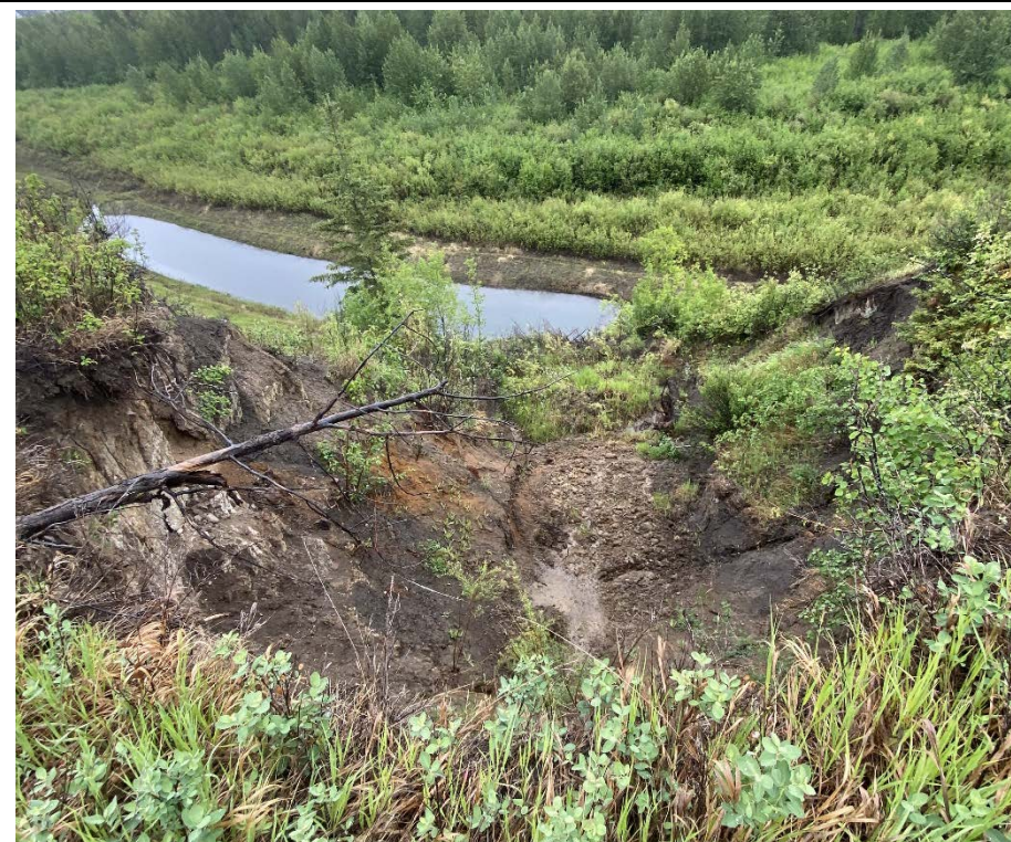
Photo 3. Looking east and downslope from the top of the main scarp of Slide 2. Ongoing erosion within the exposed and disturbed soils but no significant expansion or retrogression towards the highway since 2023. Main scarp was offset 7.6 m from the guardrail.
