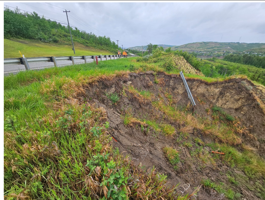
Photo 2. Looking northeast from the south side of the main scarp of Slide 1. Minor lateral expansion of the north slide flank since 2023.
