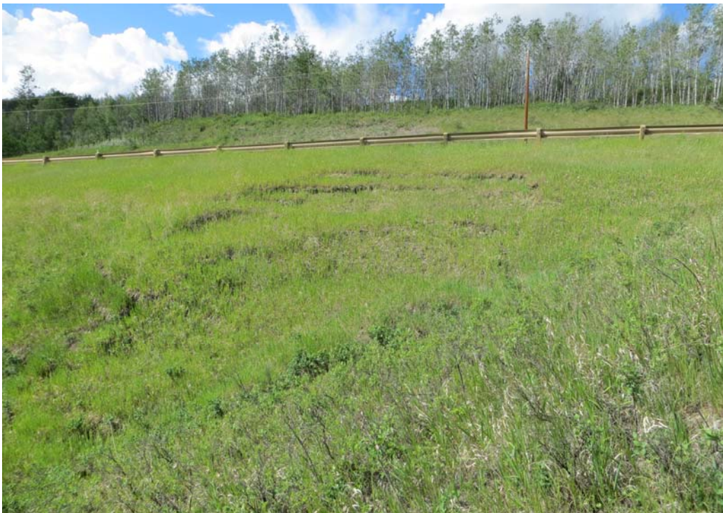
Photo 4 - Looking northwest at a slide lobe of Site A extending close to the highway.
