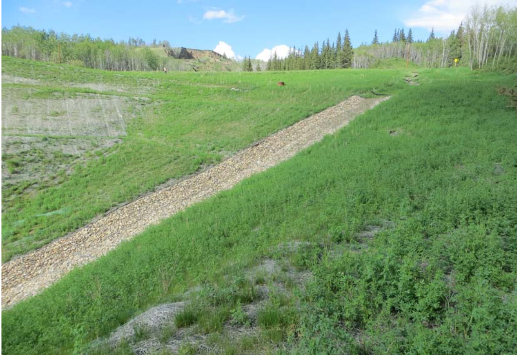
Photo 11 – Looking north up along the south embankment of Site B.
