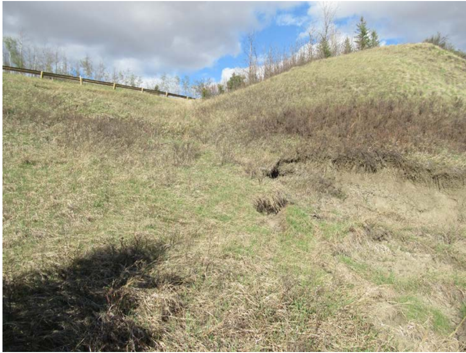
Photo 3 – Looking northwest at the slide lobe adjacent to the highway at PH77-1.
