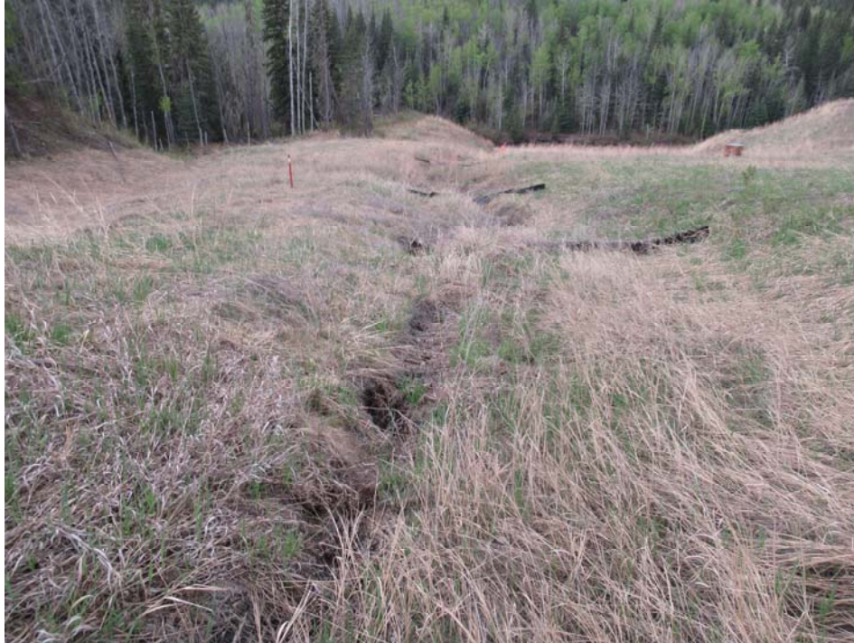
Photo 7 – Looking south along the ditch channel of PH77-2. Note the erosion, and the benched hillside to the west.
