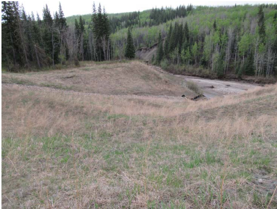
Photo 8 - Looking southeast at the culvert outlet area of PH77-2, Hines Creek.
