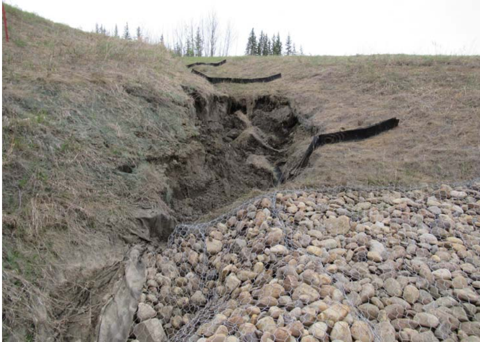
Photo 11 – Looking southeast at the erosion along the northeast ditch crotch leading to the culvert inlet area of the north embankment of PH77-2.
