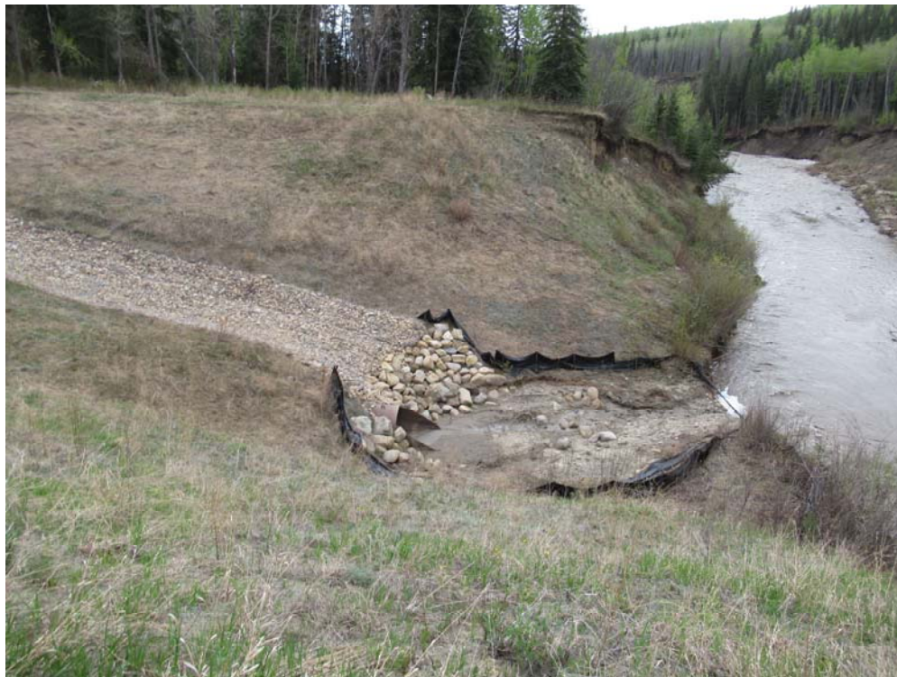
Photo 10 - Looking southeast at the culvert outlet area of PH77-2.
