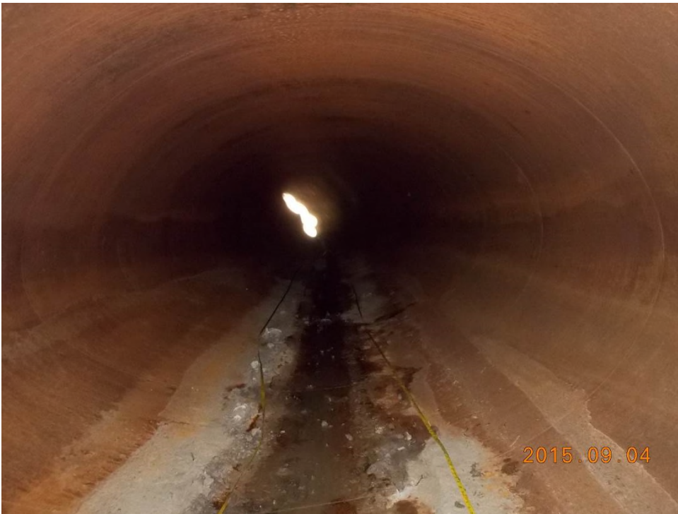
View of typical deflection looking u/s from access hole
