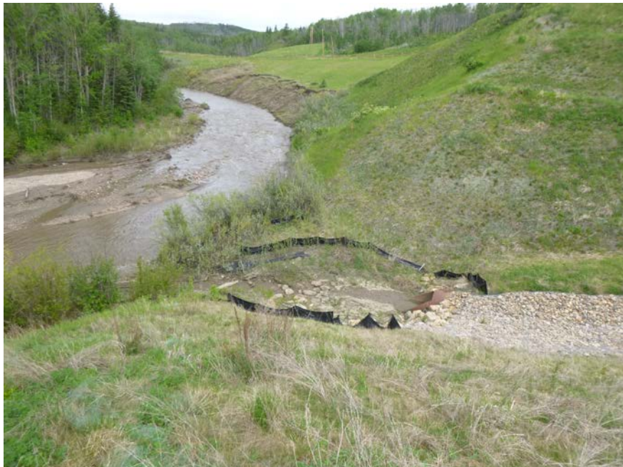
Photo 10 - Looking west at the culvert outlet area of Site 2, Hines Creek.
