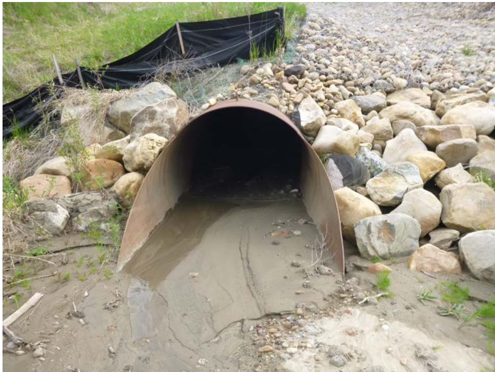
Photo 12 - Looking northeast at the culvert outlet area of Site 2.
