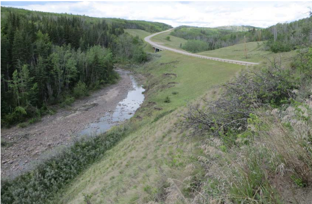
Photo 4 - Looking northwest at a slide lobe of Site 1 extending close to the highway.
