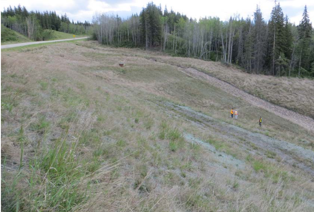
Photo 11 – Looking east along the upper south embankment of Site 2.
