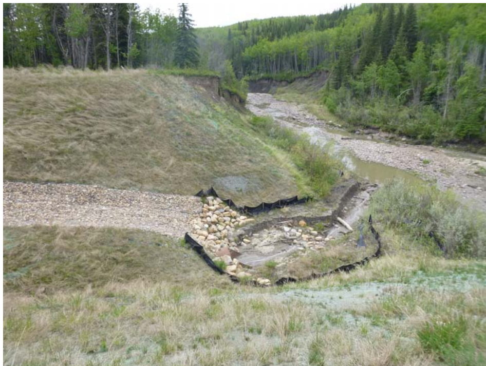
Photo 10 - Looking east at the culvert outlet area of Site 2, Hines Creek.
