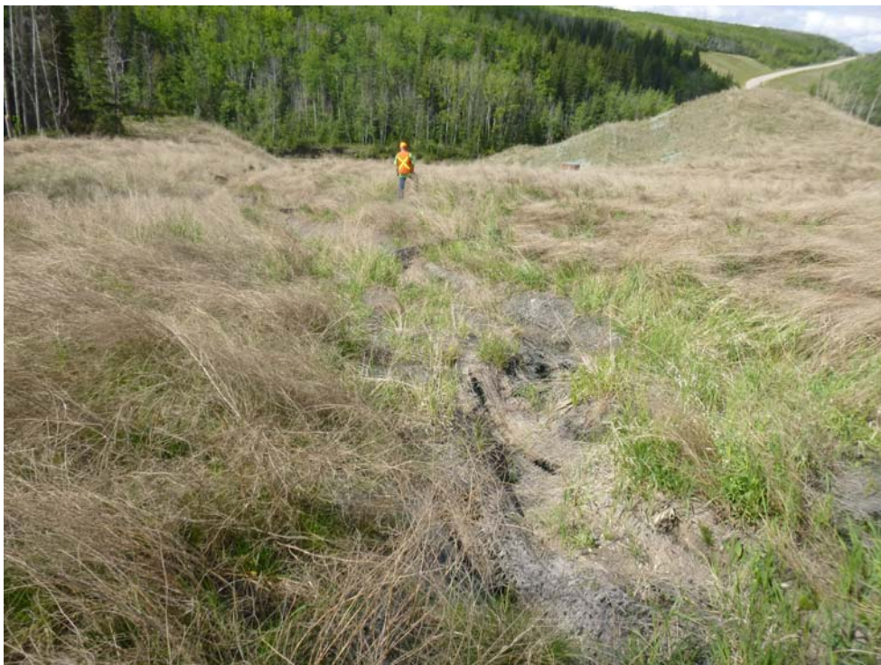
Photo 8 - Looking at the surface erosion through the existing erosion control soil covering and ditch barriers on the south embankment of Site 2.
