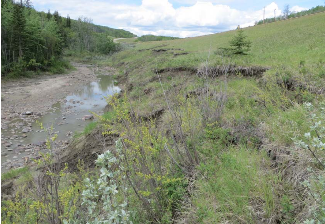
Photo 3 – Looking west along the slide scarp adjacent to the Creek at Site 1.
