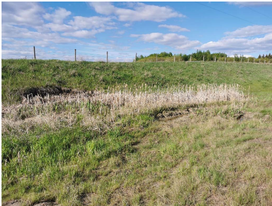
Photo 6 – Looking northeast at spring observed in backslope east of the site. Cattails and ponded water present in the ditch.
