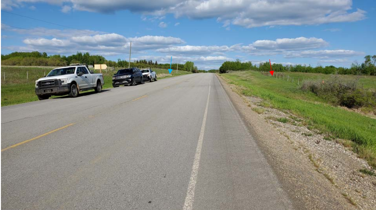
Photo 1 – Looking east along slight rise in the highway as there is a low backslope cut on the north side behind the trucks. The cattails are roughly where the seep was observed (blue arrow). The second groundwater well was on the higher ground to the south (red arrow)
