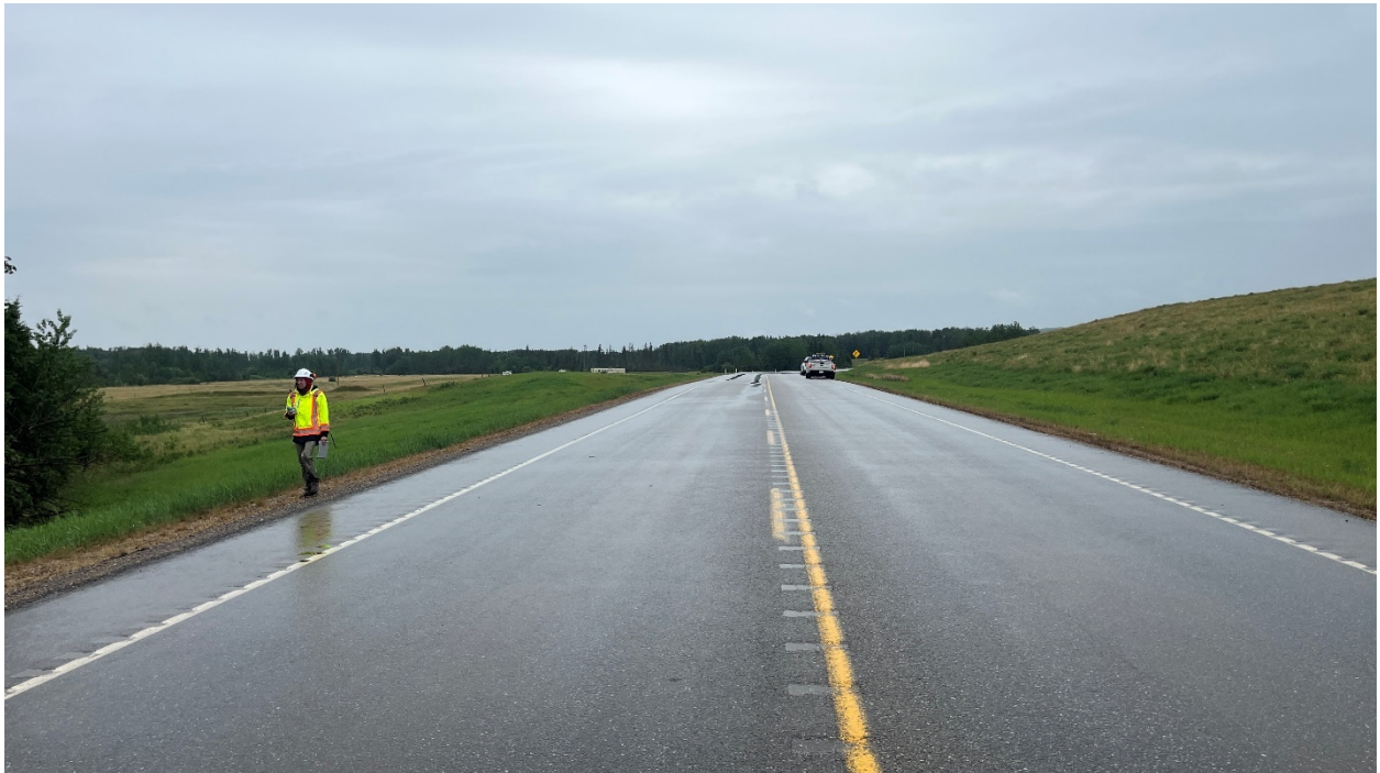
Photo 2 – Looking west along Hwy 679 above the slide site.
