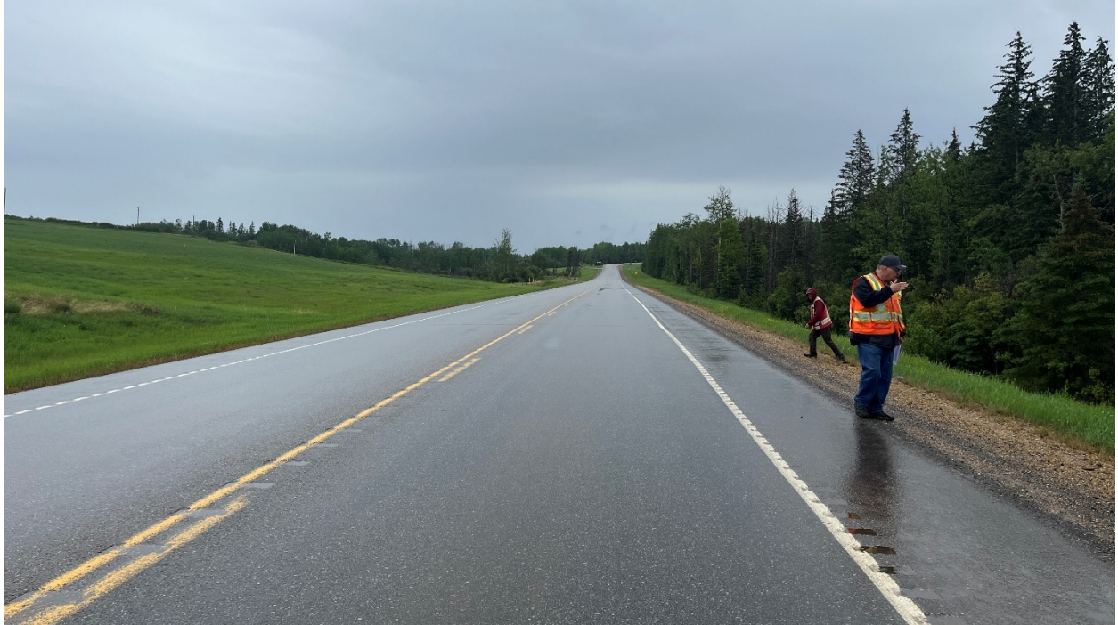
Photo 1 – Looking east along Hwy 679 above the slide site towards the intersection at Hwy 750.
