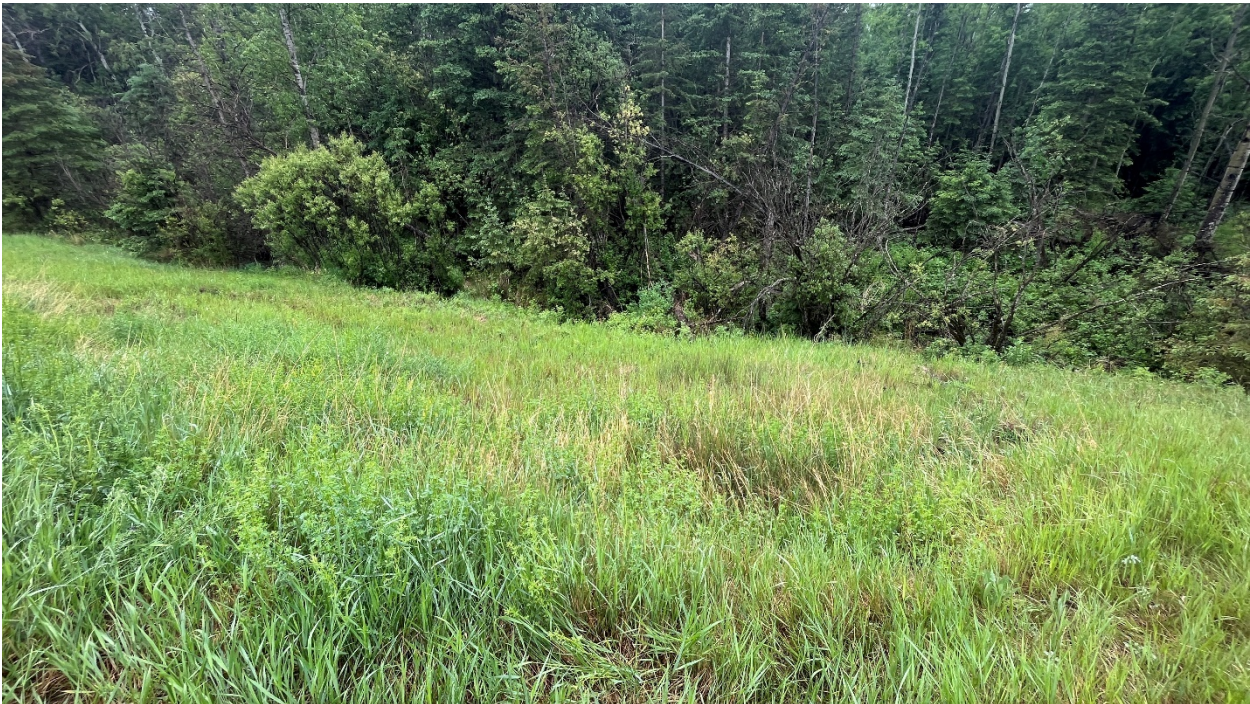
Photo 4 – Looking south down along the slide from the edge of the highway.
