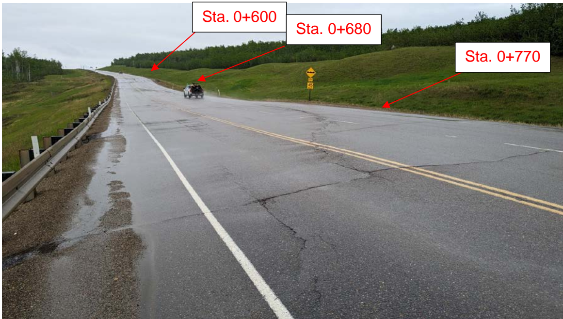
Photo 3 – Looking east where the main scarps cross the highway at three locations.
