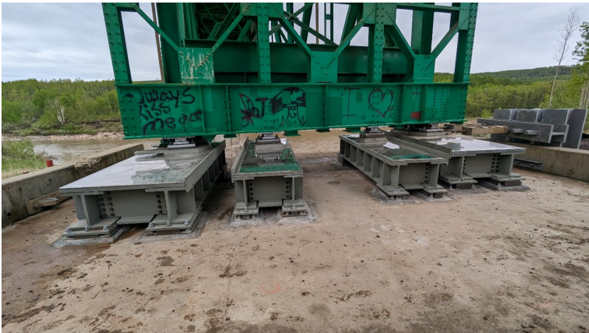
Photo 6 – New slide plates installed at Pier 1.
