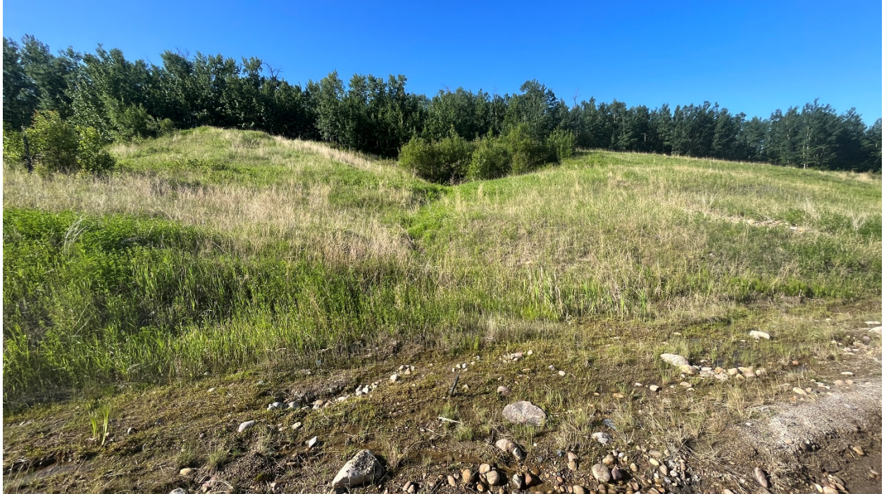
Photo 5: Lower portion of the slope at toe of Slump B becoming vegetated since the 2019 grading work.
