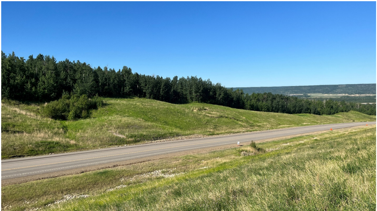
Photo 6: Looking southwest at Slump D.
