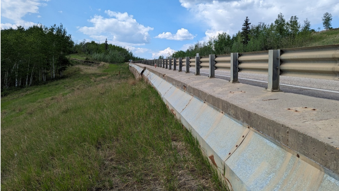
Photo 1 – Looking northwest along the pile wall.
