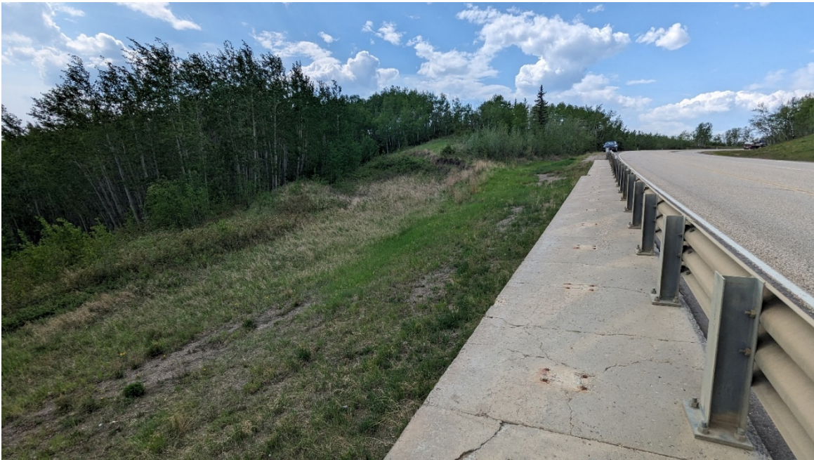
Photo 8 – Looking west at graben block northwest of the wall, which appears to have become re-activated.
