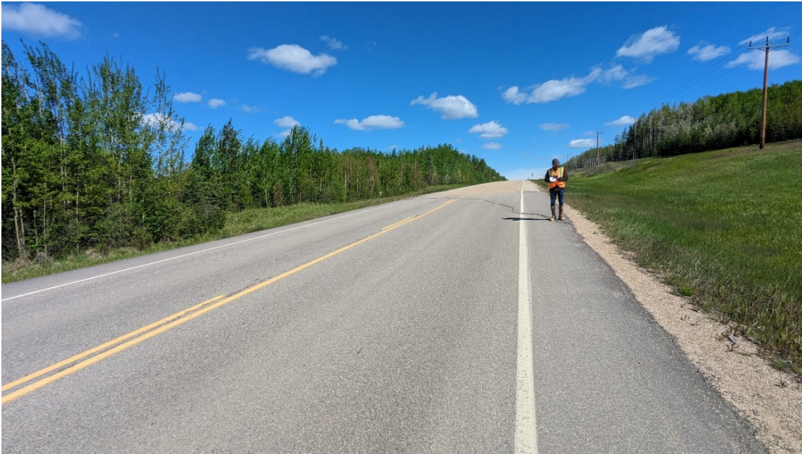
Photo 3: Looking north at hump over main scrap crack at north end of the site.
