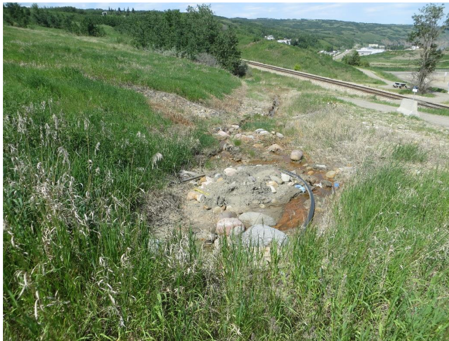
Photo 7. Looking northeast at the outlet of the twin culverts.
