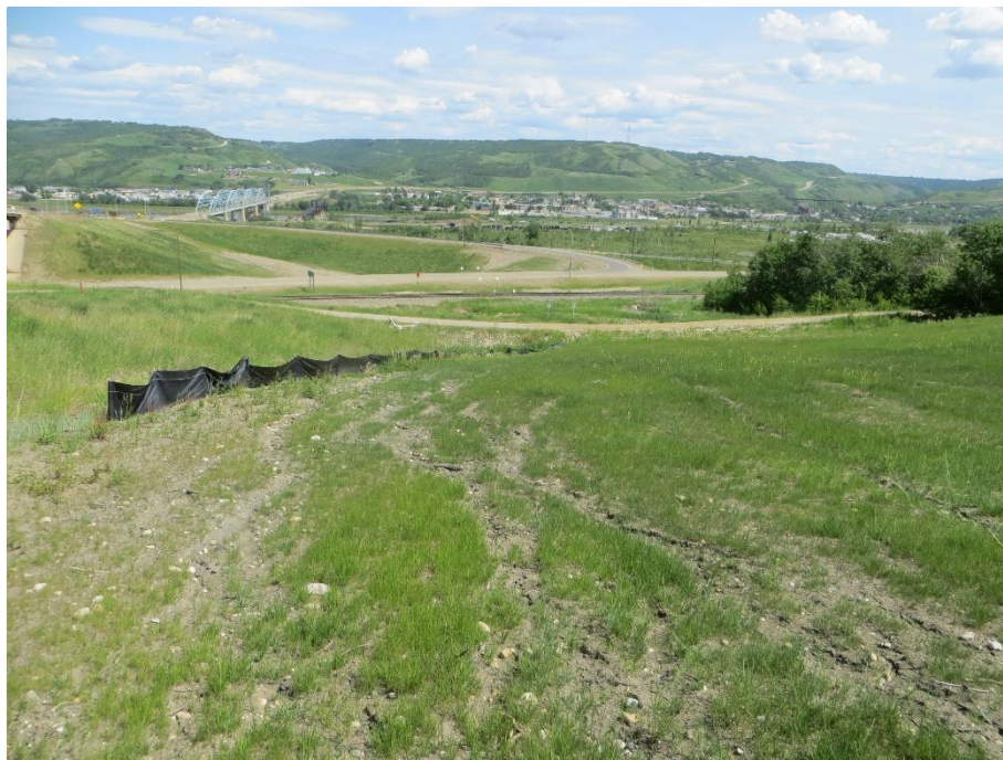
Photo 16. Looking northeast at the area that was regraded as part of the new storm utility pipe installation in 2016.
