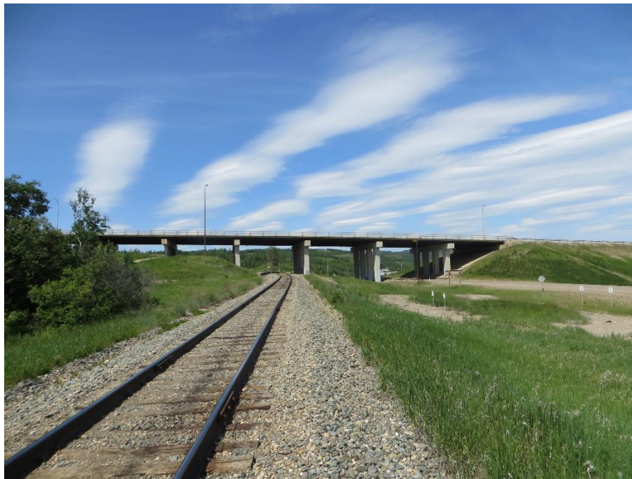
Photo 1. Looking northwest at Shafstbury Trail overpass. CN has cleaned the ditch on the west side of the railway and have re-ballasted the tracks.
