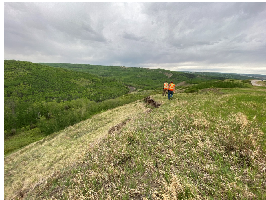
Photo 70-09. Looking west from the east end of the active landslide scarp developing west of the pile wall (34+050). There was a more visible scarp with increased dropdown (up to 1.5 m deep) and the tension cracks have extended and opened up further relative to the 2023 condition.
