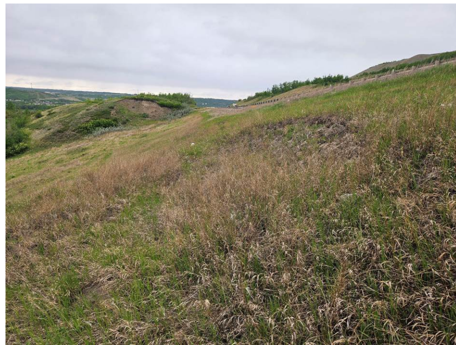
Photo 61-03. Looking west towards the shallow slide scarp approximately 10 m below the highway (36+350). Some minor movement within the slide mass but scarp is vegetated and there were no major visible changes since 2022.
