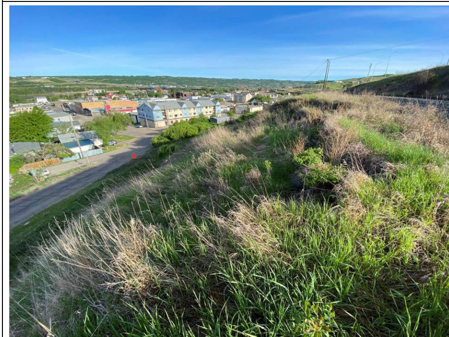
Photo 61-13. Intermittently active shallow sliding occurring downslope of the CN tracks near KM 37+300. Main scarp was offset approximately 35 m from southwest pavement edge.
