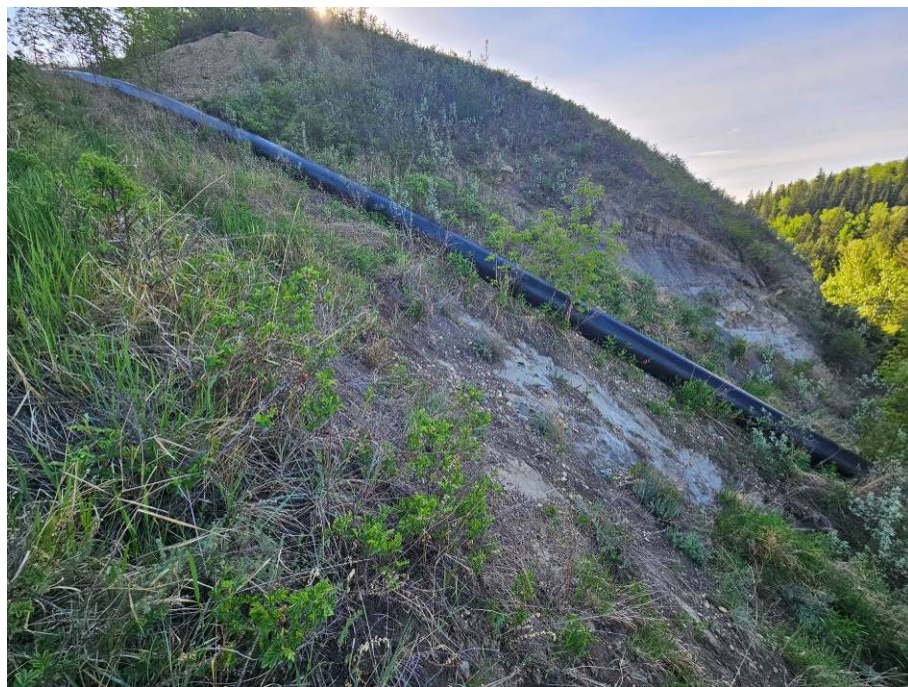
Photo 61-10. View looking southeast at ongoing erosion of fill area around the lower segment of the elephant trunk drain (km 36+475). Erosion and vegetation disturbance was slightly worse relative to the 2022 condition.
