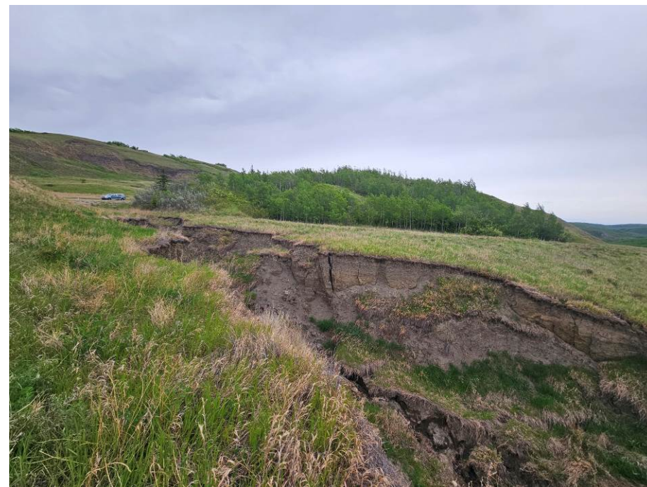
Photo 60-06. Looking north towards expanded gully erosion downstream from km 36+050. Ongoing erosion and collapse of the near vertical gully sidewalls.
