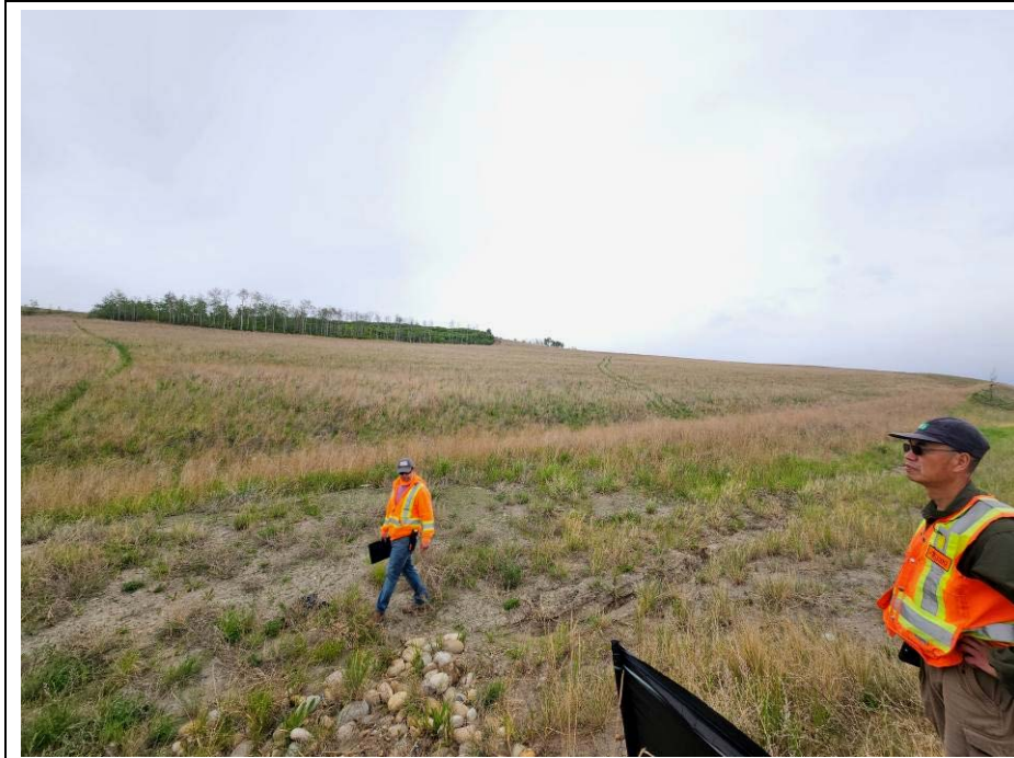
Photo 59-03. Looking northeast at the borrow area upslope of the highway between approximately 34+700 and 35+200. Slope was well vegetated with minor track erosion from off-highway vehicles. No stability issues were apparent.
