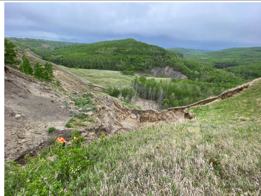
Photo 2-16. View east of the expanded erosion gully below the hanging trunk pipe breach.
