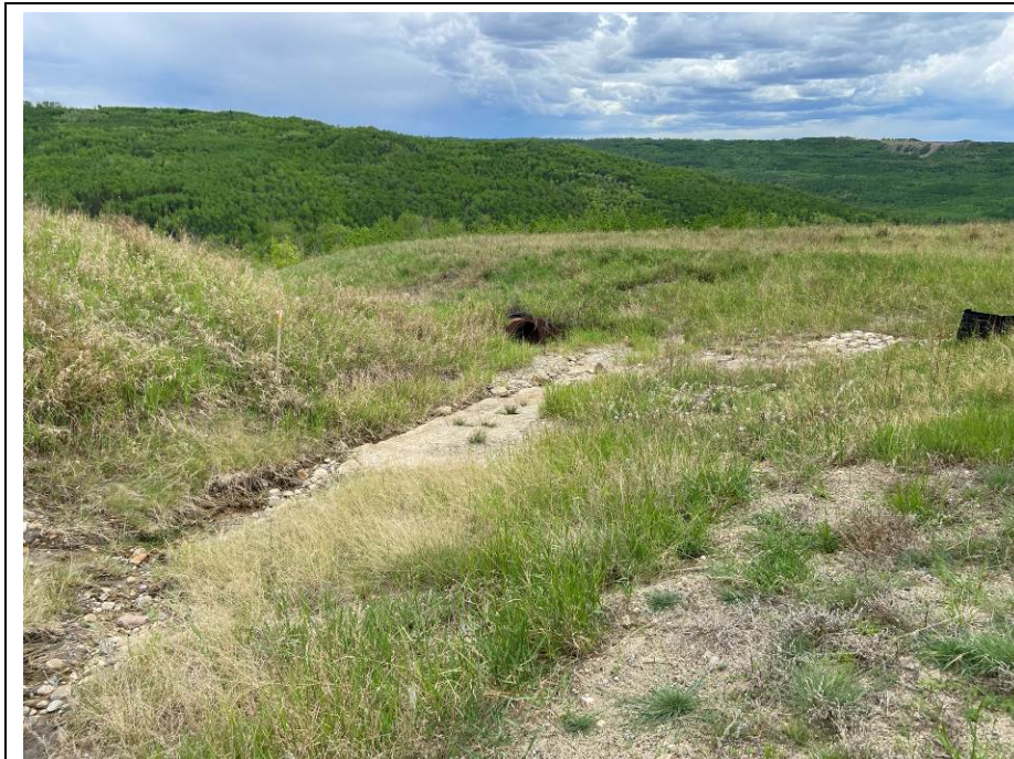
Photo 2-09. Looking south at trunk drain inlet at km 33+715. Minor gully erosion upstream of inlet between the ditch repairs but no major change from the 2022 condition.
