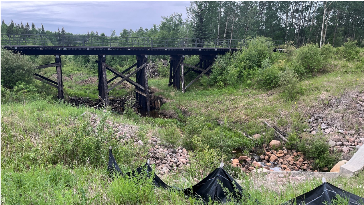
Photo 12 – Looking south at culvert inlet and adjacent rail bridge.
