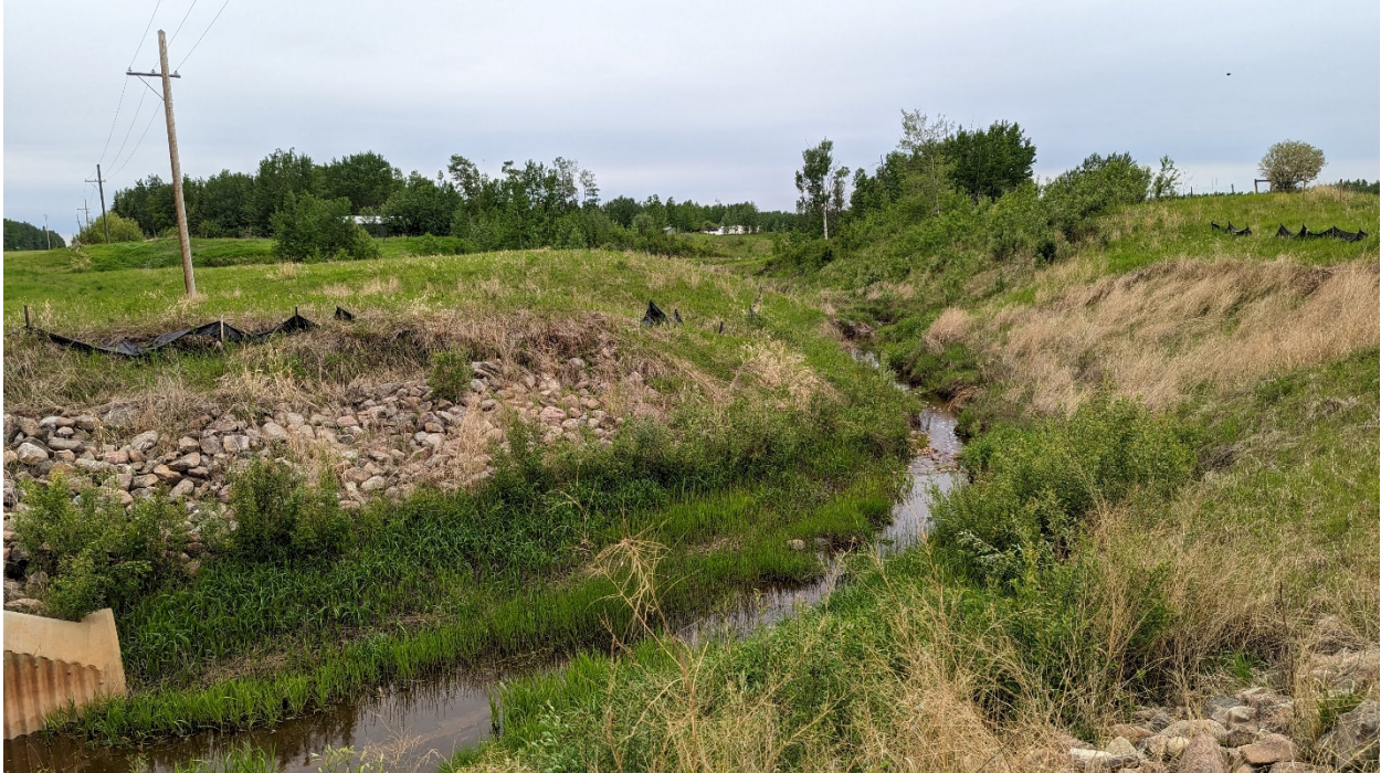
Photo 7 – Looking north (downstream) along the creek. There is minor slumping at the top of the riprap on the west (left) side and a larger slump further downstream on the right (east) side.
