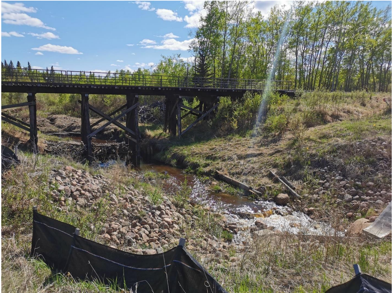
Photo 13 – Looking south at culvert inlet and adjacent rail bridge.
