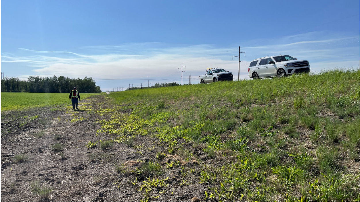
Photo 3 – Looking west along south side slope of highway embankment.
