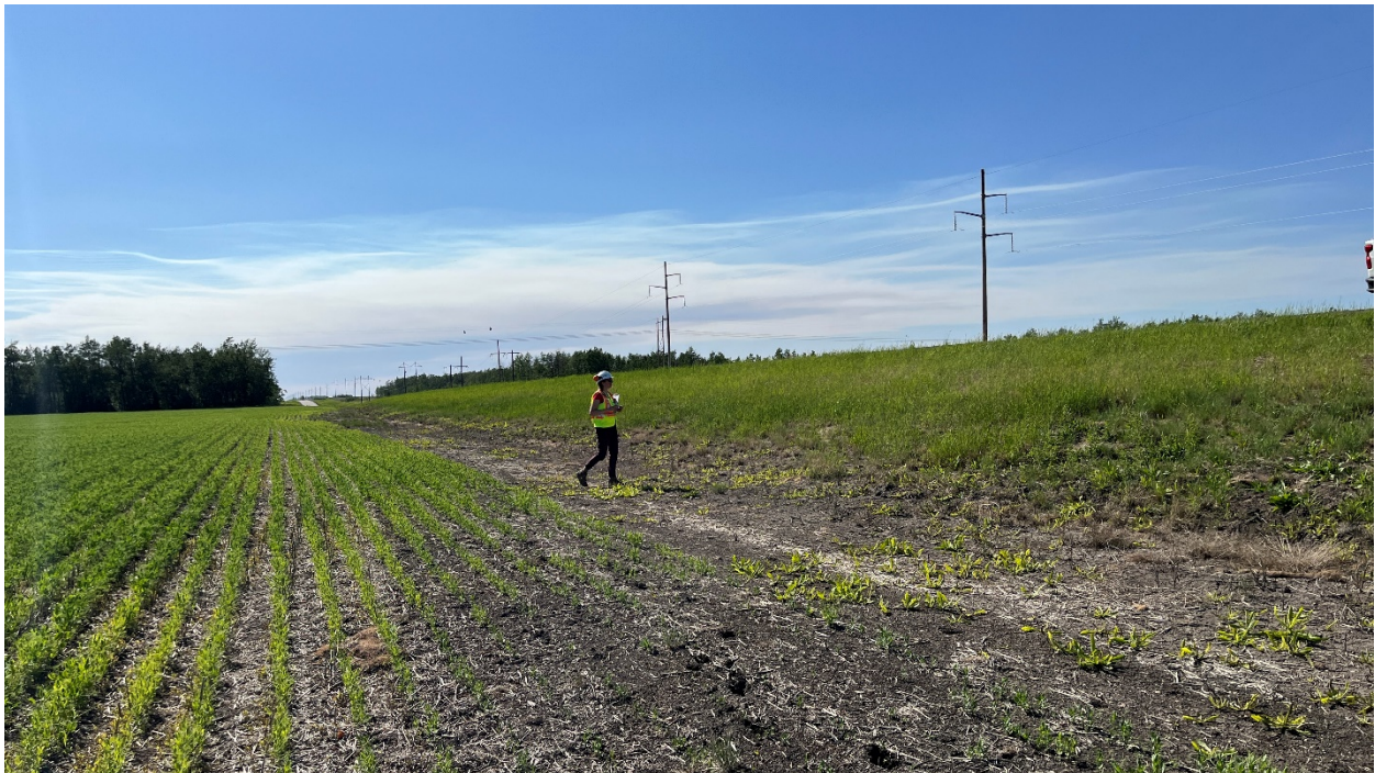
Photo 4: Looking west along south ditch where TRM was installed.
