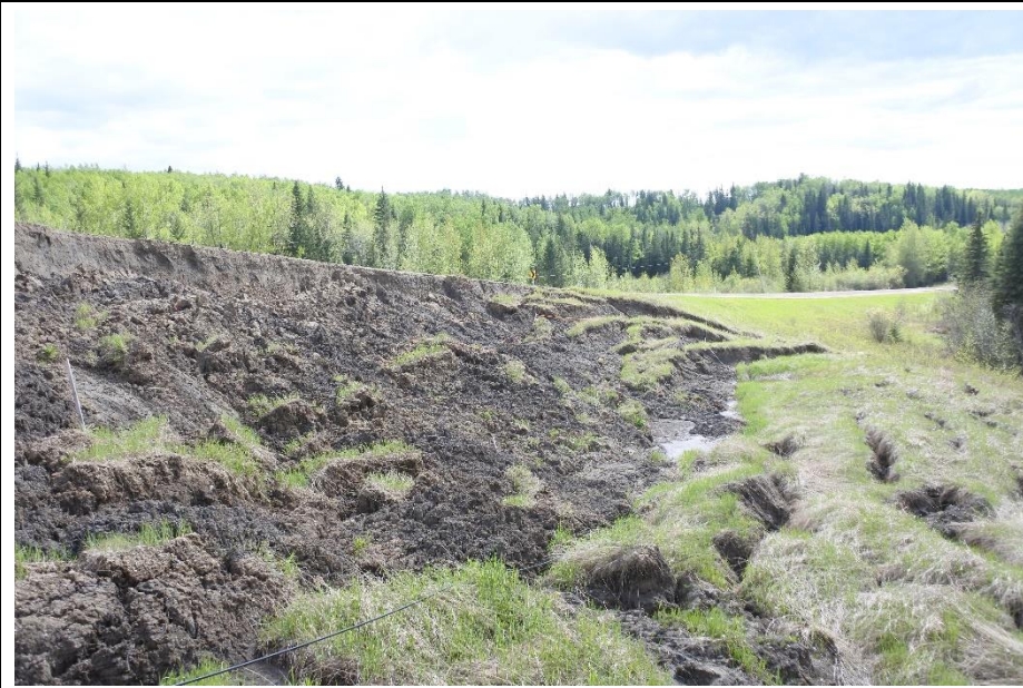
Photo 7. Looking south at the back scarp and wet slide mass.
