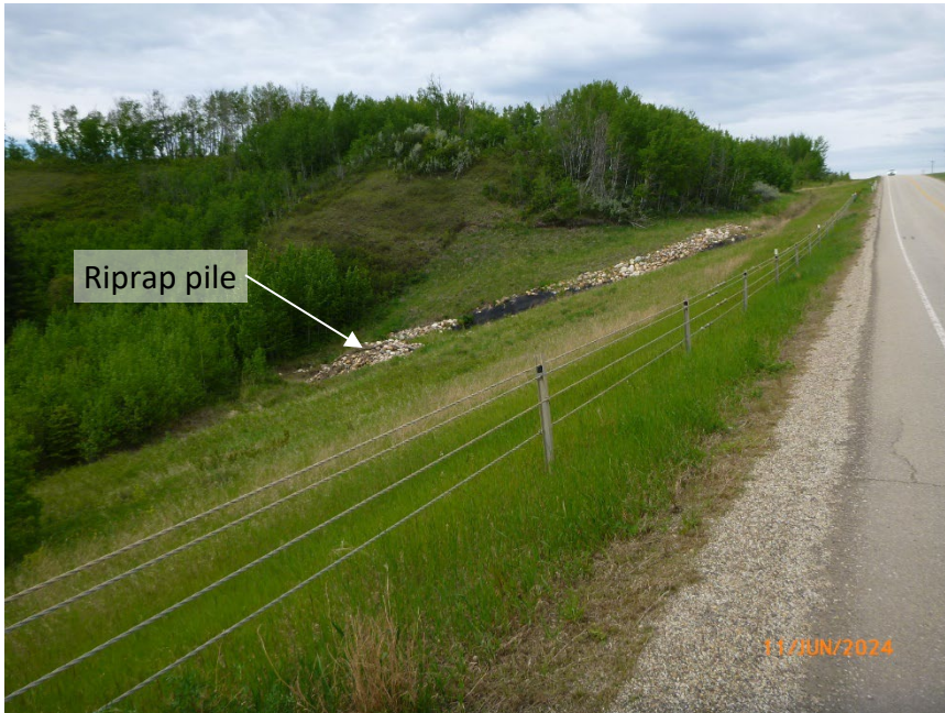
Photo 2 Displaced riprap deposited in pile near bottom of ditch channel. Note exposed geotextile is damaged and undermined. Photo taken June 11, 2024, facing southwest.
