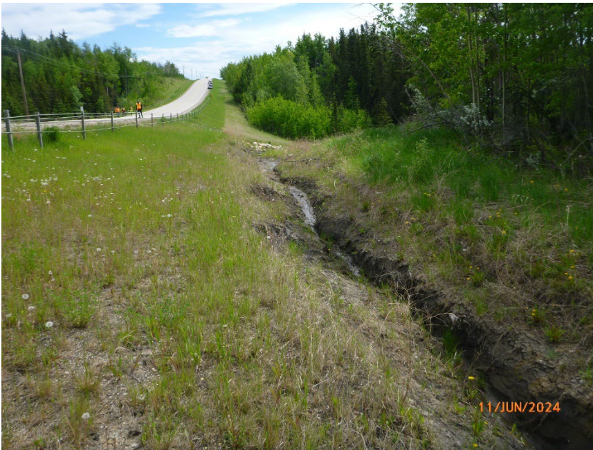
Photo 4 Channel eroded into bottom of ditch channel on west side of Hwy 733:02. Note guardrail located downslope of pavement edge. Photo taken June 11, 2024, facing south.
