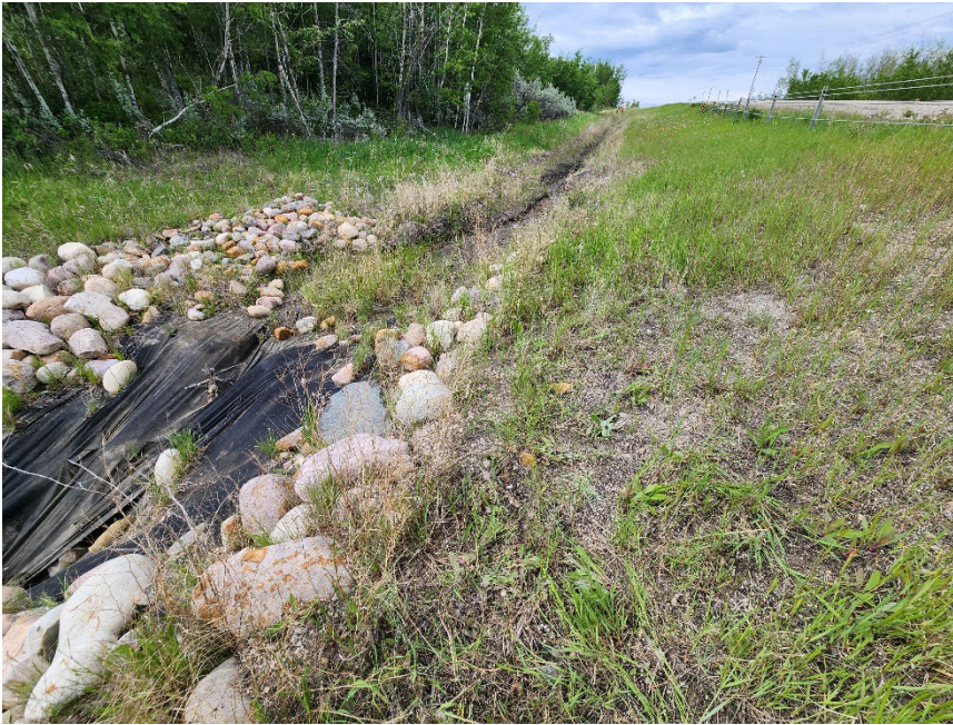
Photo 4 Channel eroded into bottom of ditch channel on west side of Hwy 733:02. Note guardrail located downslope of pavement edge. Photo taken June 11, 2024, facing south.
