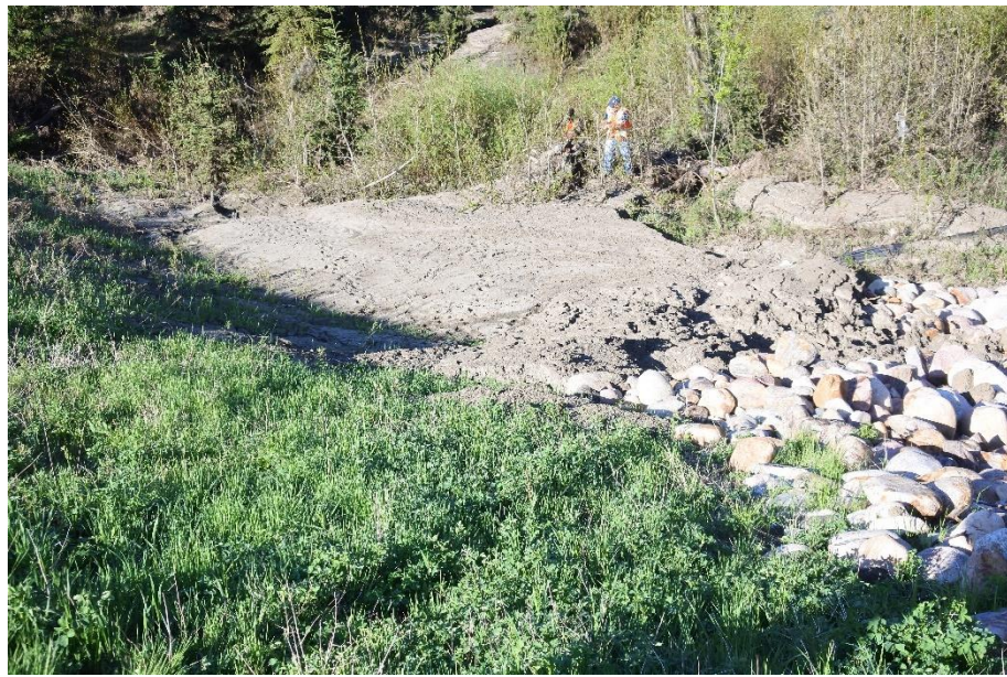
Photo 7. Looking southwest at the accumulation of mud and silt near the toe of the embankment slope above the creek.
