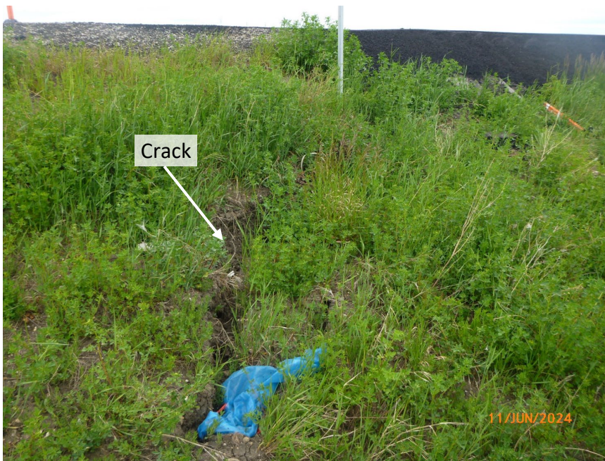
Photo 4 Cracking along south slope of Hwy 674:02 embankment. Photo taken June 11, 2024, facing north.
