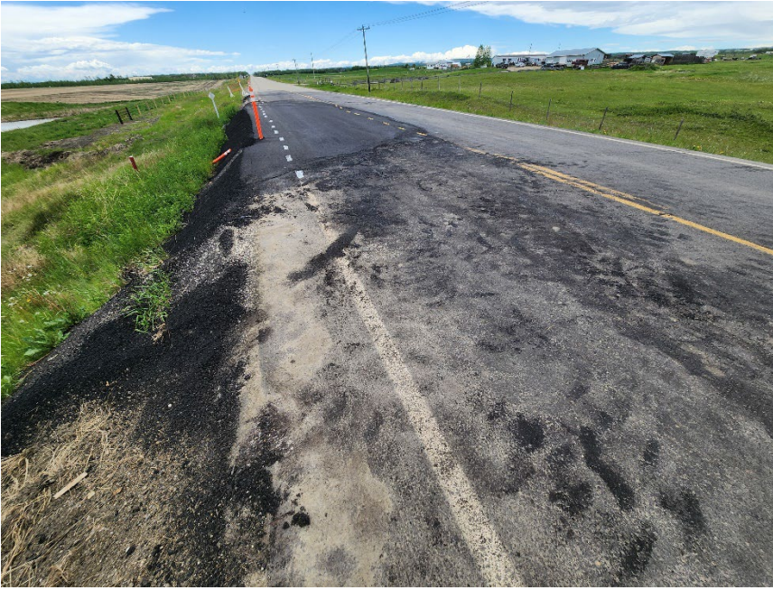
Photo 2 Cracking and settlement in eastbound lane of Hwy 674:02. Note near-vertical edge and height of exposed pavement. Photo taken June 11, 2024, facing northeast.
