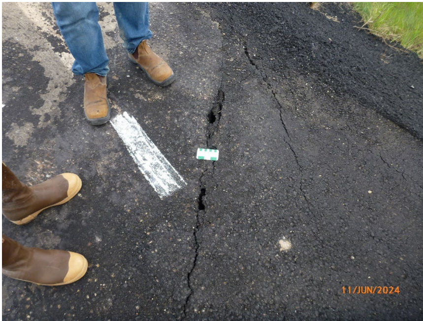
Photo 4 Cracking along south slope of Hwy 674:02 embankment. Photo taken June 11, 2024, facing north.
