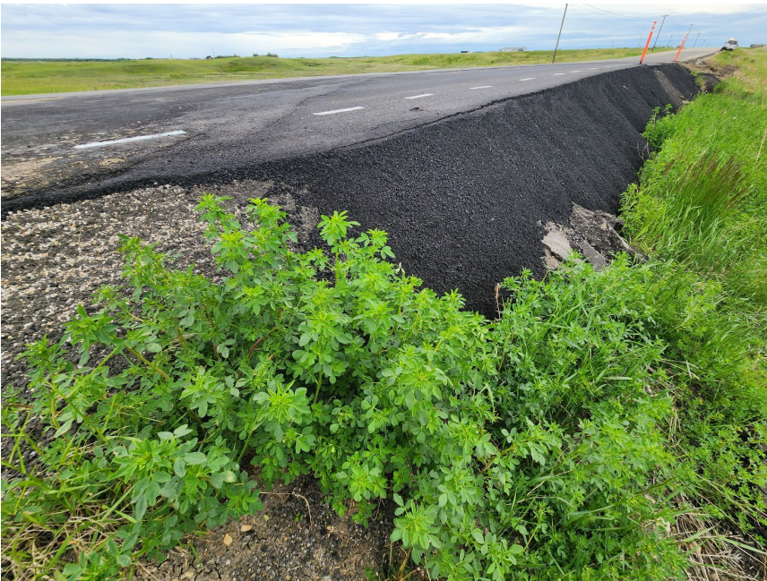
Photo 2 Cracking and settlement in eastbound lane of Hwy 674:02. Note near-vertical edge and height of exposed pavement. Photo taken June 11, 2024, facing northeast.
