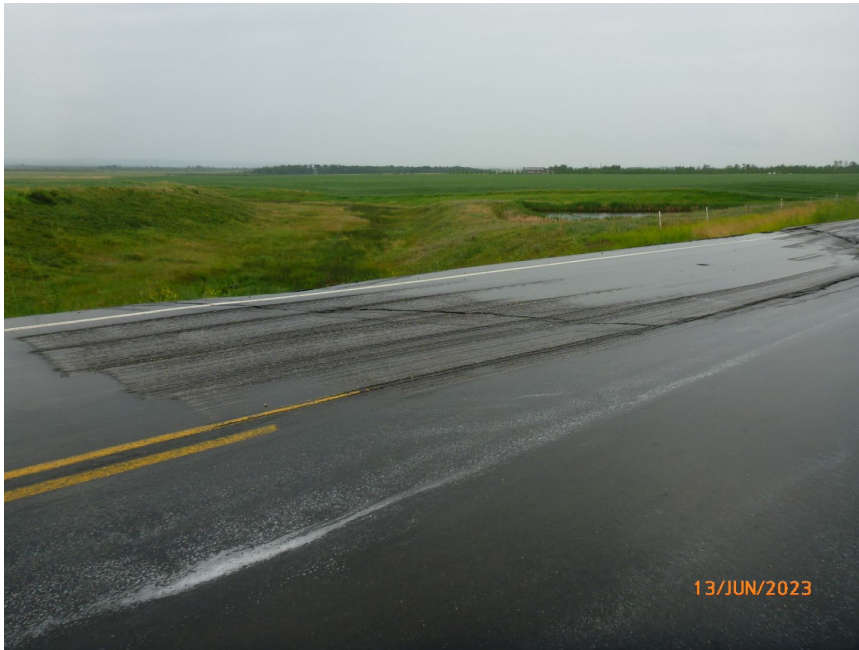
Photo 2 Cracking and settlement along slide headscarp in south (eastbound) lane of Hwy 674:02. Photo taken June 13, 2023, facing west.
