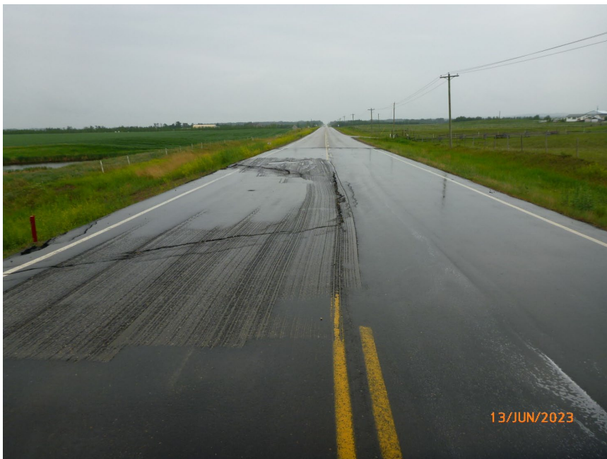
Photo 2 Cracking and settlement along slide headscarp in south (eastbound) lane of Hwy 674:02. Photo taken June 13, 2023, facing west.
