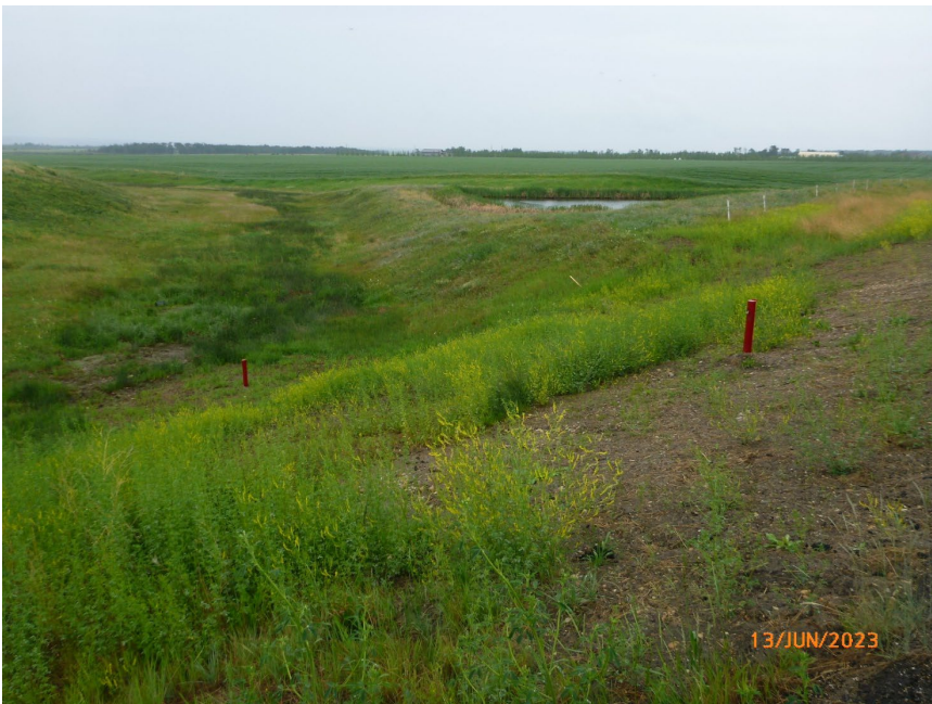
Photo 4 Slope and toe area of slide on south side of Hwy 674:02 embankment. Note pond water in dug out southwest of highway embankment and slide. Photo taken June 13, 2023, facing southwest.
