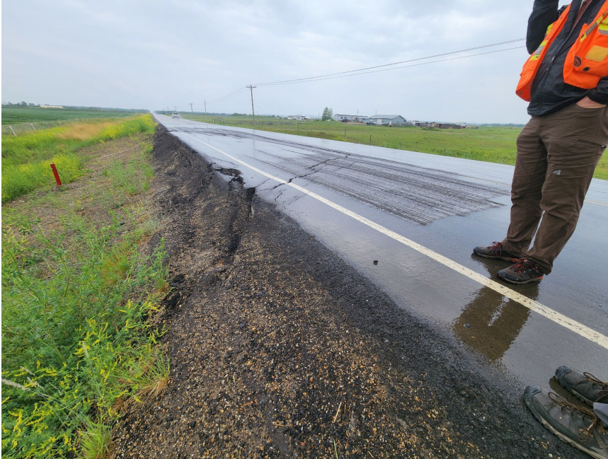
Photo 4 Slope and toe area of slide on south side of Hwy 674:02 embankment. Note pond water in dug out southwest of highway embankment and slide. Photo taken June 13, 2023, facing southwest.
