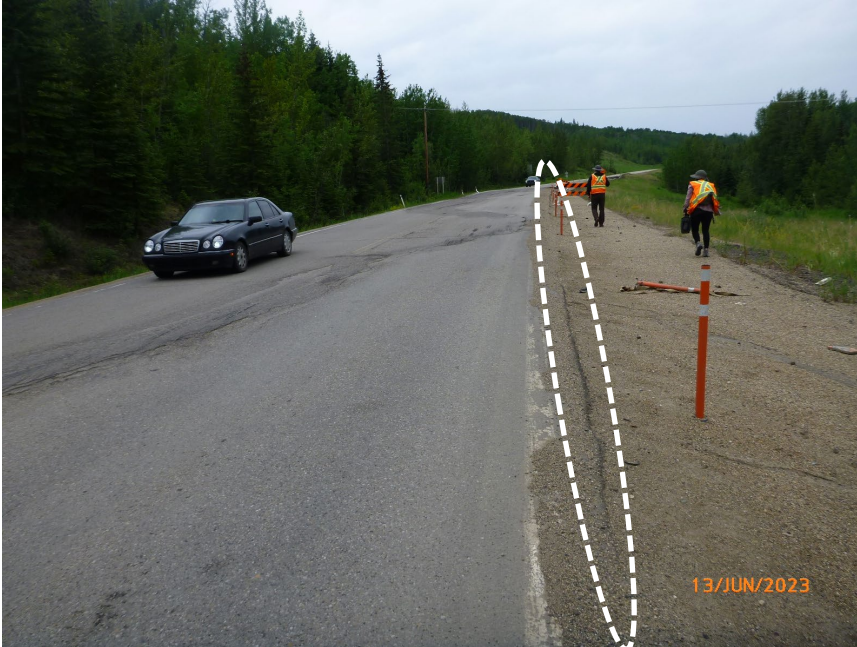
Photo 7 Cracking and settlement in westbound (north) lane of Hwy 666:02 at GP016-2 (lower) site. Note drop in pavement along slide scarp. Photo taken June 13, 2023, facing southwest.
