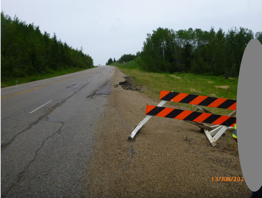
Photo 15 Pavement breaking away highway along westbound (north) shoulder of Hwy 666:02 at GP016-3 (upper) site. Photo taken June 13, 2023, facing southwest.
