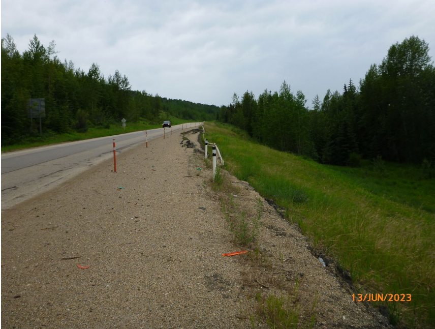
Photo 9 Pavement breaking away highway along westbound (north) shoulder of Hwy 666:02 at GP016-2 (lower) site. Note guardrail deflected and below top of pavement. Photo taken June 13, 2023, facing northeast.
