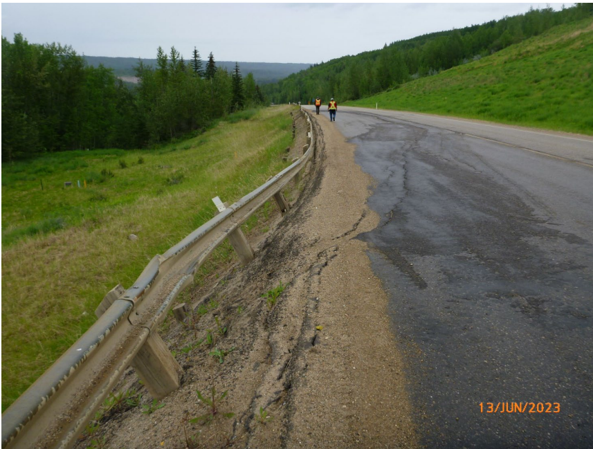
Photo 11 Cracking and settlement in westbound (north) lane of Hwy 666:02 at GP016-1 (middle) site. Note guardrail deflected at a similar level as top of pavement. Photo taken June 13, 2023, facing northeast.
