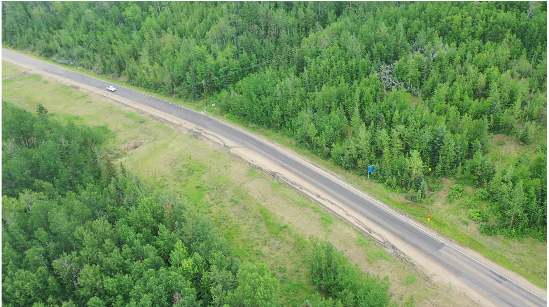
Photo 2 Overview of GP016-2 (lower) site. Note pavement patches, and cracking and settlement along both lanes of Hwy 666:02. Photo taken June 13, 2023, facing southeast.
