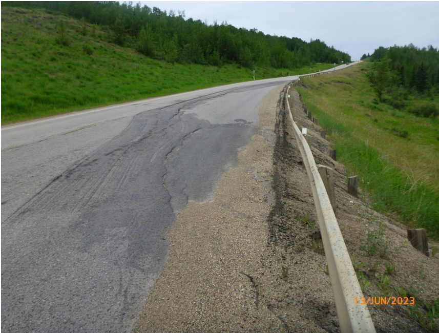
Photo 11 Cracking and settlement in westbound (north) lane of Hwy 666:02 at GP016-1 (middle) site. Note guardrail deflected at a similar level as top of pavement. Photo taken June 13, 2023, facing northeast.
