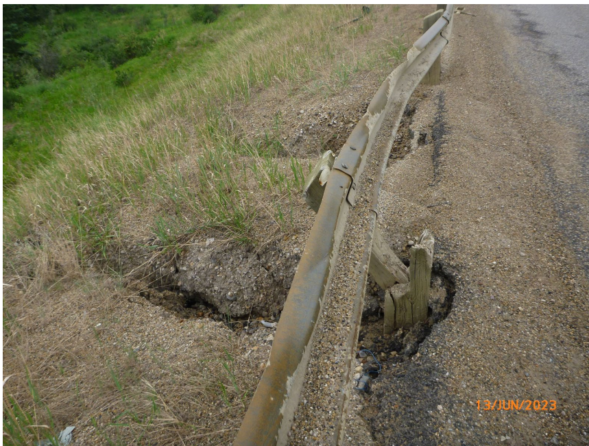
Photo 13 Erosion at WP316 due to surface water flow over edge of pavement. Note guardrail also deflected and post is damaged. Photo taken June 13, 2023, facing southwest.
