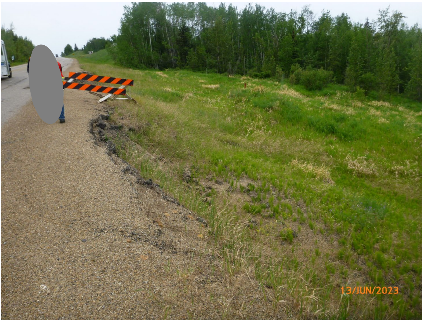
Photo 15 Pavement breaking away highway along westbound (north) shoulder of Hwy 666:02 at GP016-3 (upper) site. Photo taken June 13, 2023, facing southwest.
