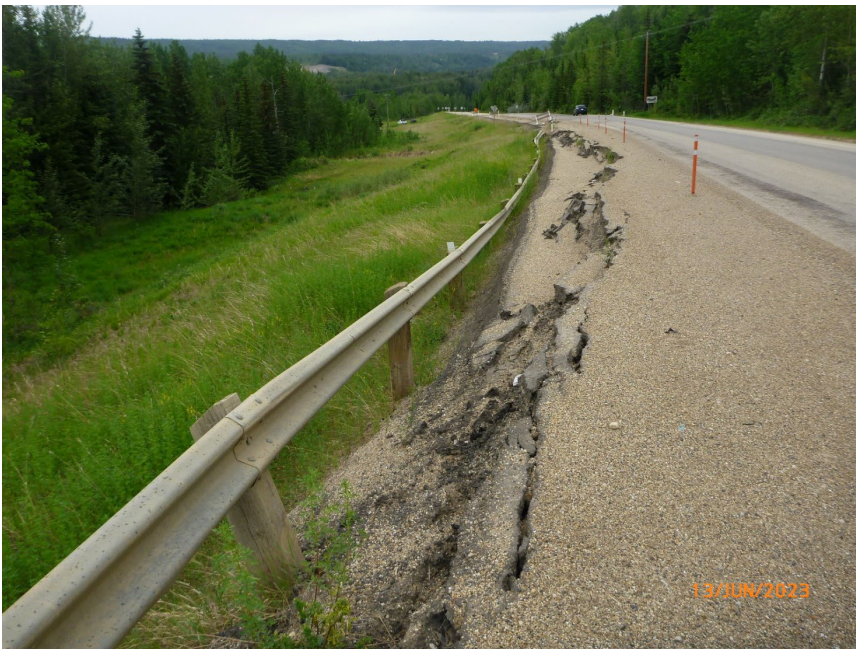
Photo 9 Pavement breaking away highway along westbound (north) shoulder of Hwy 666:02 at GP016-2 (lower) site. Note guardrail deflected and below top of pavement. Photo taken June 13, 2023, facing northeast.
