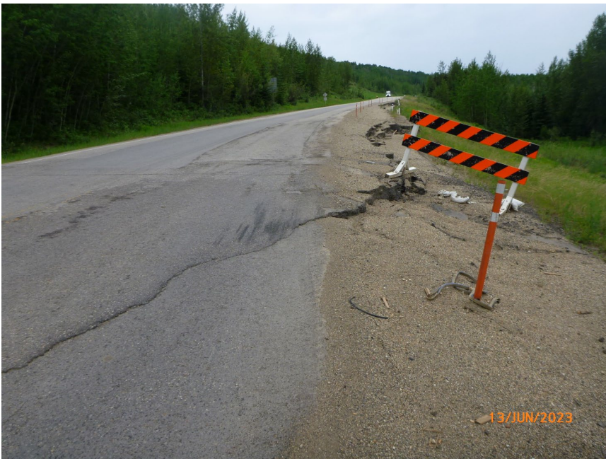
Photo 7 Cracking and settlement in westbound (north) lane of Hwy 666:02 at GP016-2 (lower) site. Note drop in pavement along slide scarp. Photo taken June 13, 2023, facing southwest.
