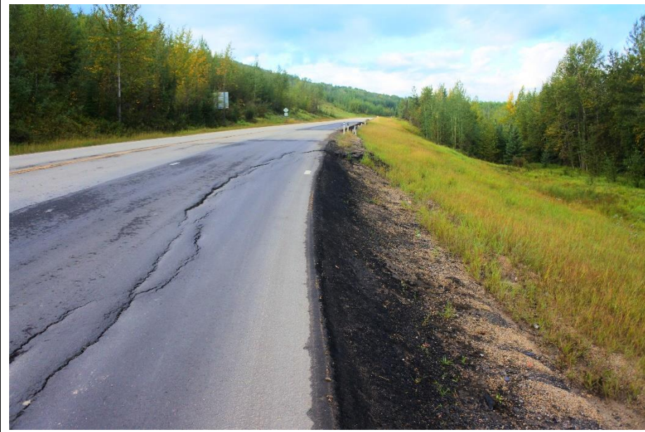
Photo 6. Looking southwest along Hwy 666 at west portion Lower Valley Landslide (Site 2). The scarp has a 0.3 m drop in the WBL shoulder.
