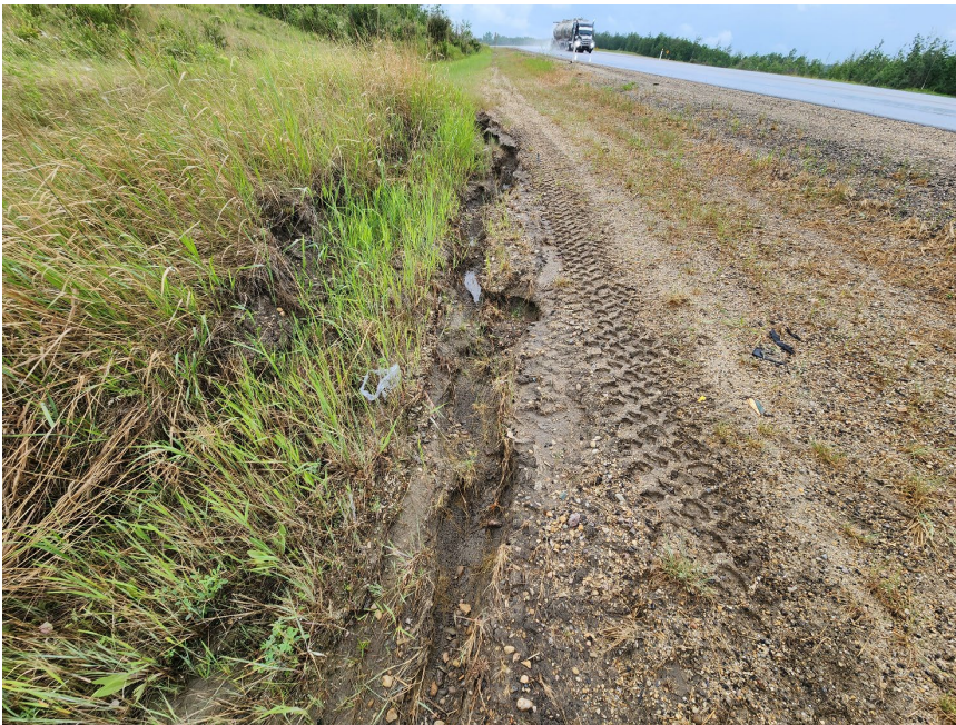
Photo 6 Erosion along toe of backslope and toe roll shown in previous photo near WP317. Photo taken June 13, 2023, facing southwest.
