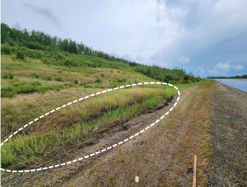
Photo 6 Erosion along toe of backslope and toe roll shown in previous photo near WP317. Photo taken June 13, 2023, facing southwest.
