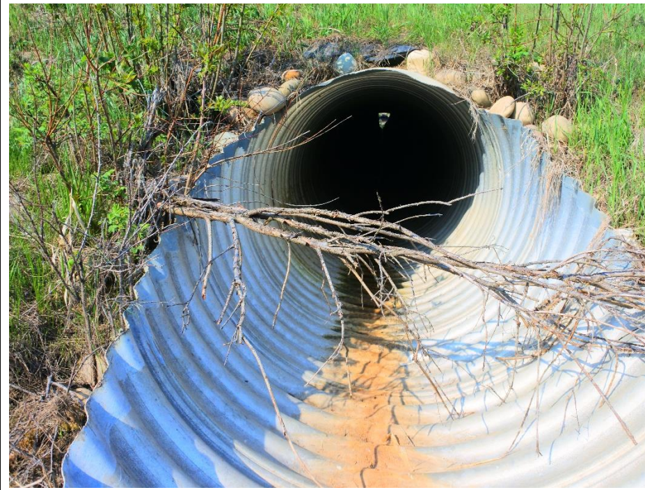
Photo 8. Looking southwest at culvert inlet.
