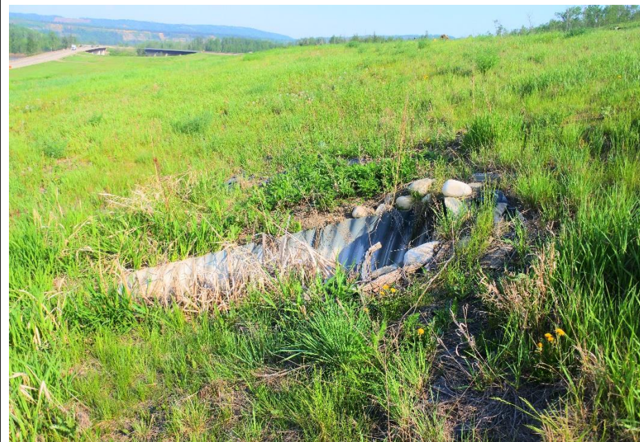
Photo 4. Looking northwest at 1200 mm diameter CSP culvert outlet.
