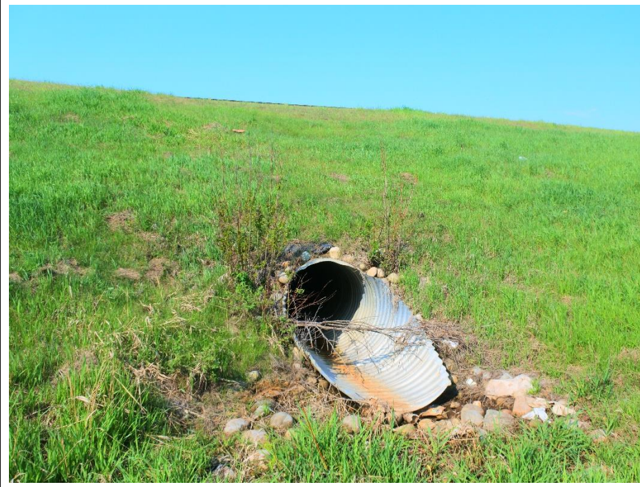
Photo 9. Looking west at culvert inlet.
