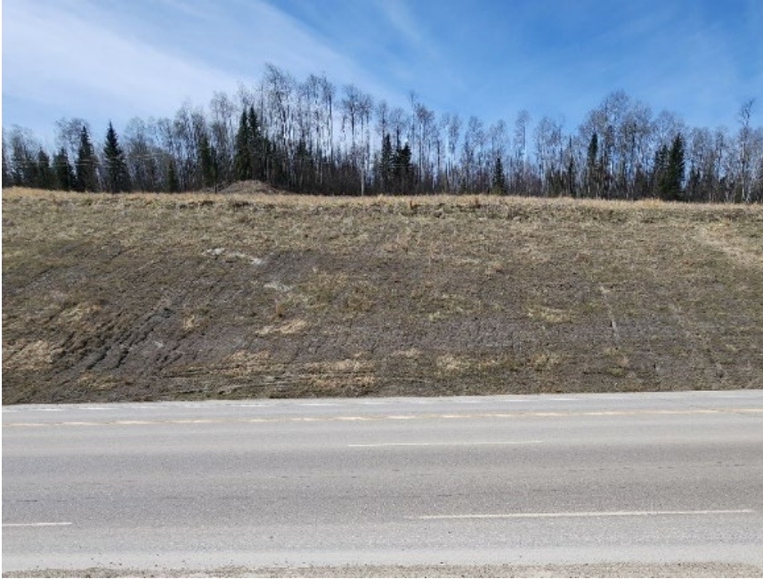
Photo 7 Erosion and seepage on backslope. Photo taken May 9, 2024, facing west.
