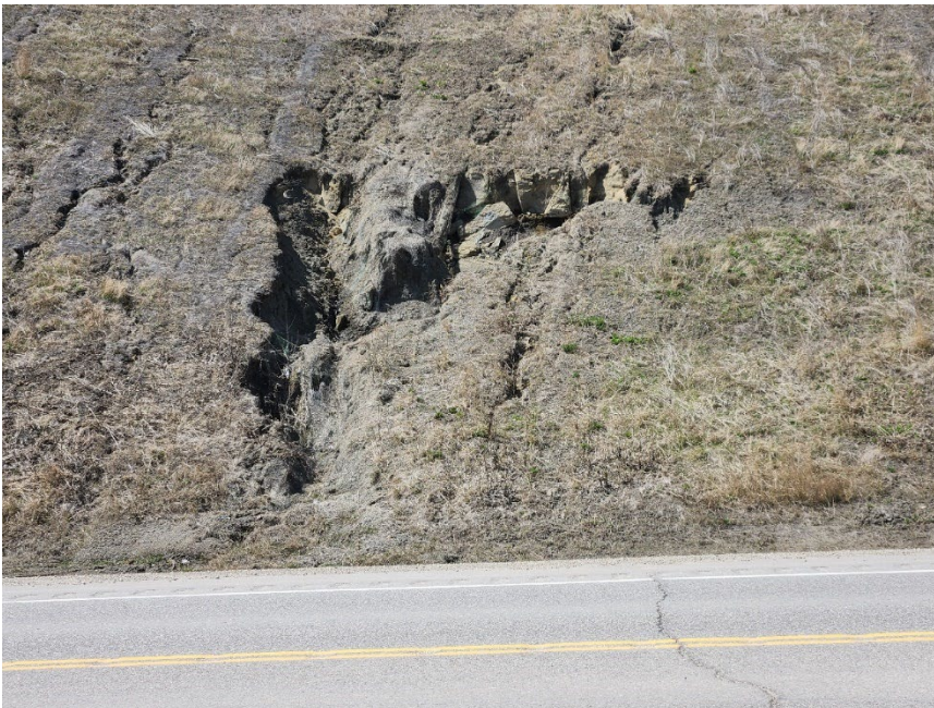
Photo 7 Erosion and seepage on backslope. Photo taken May 9, 2024, facing west.
