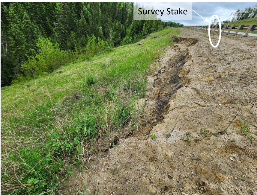
Photo 6 Slope failure and slide scarps between Hwy 40:38 and Roseham Creek. Note rill erosion on upper portion of slope (unvegetated gravelly material) and reference/survey stake with flagging (circled in white) to monitor retrogression of slide scarp. Photo taken June 11, 2024, facing south.
