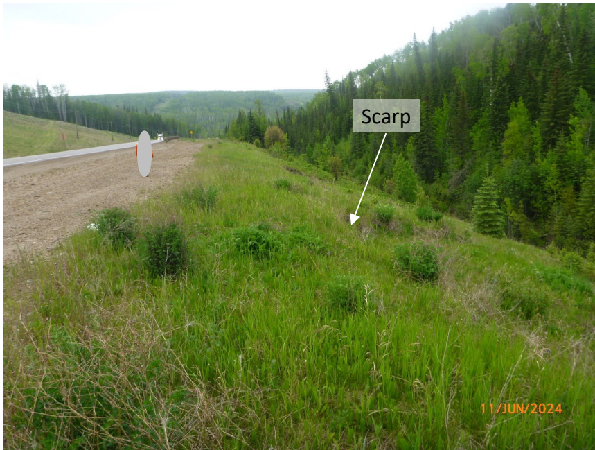
Photo 2 Slope failure and slide scarps between Hwy 40:38 and Roseham Creek. Photo taken June 11, 2024, facing north.
