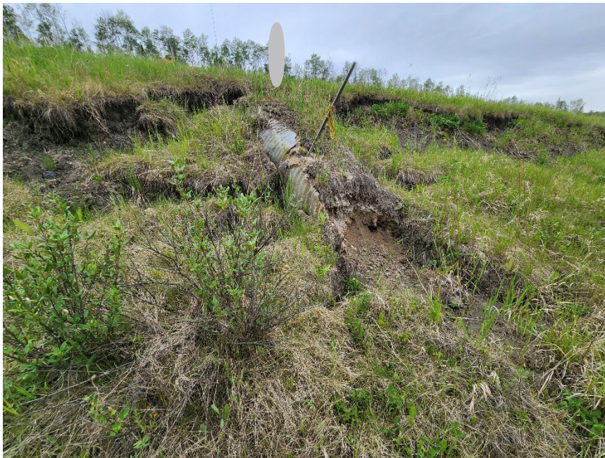
Photo 4 Culvert outlet on east side of Hwy 40:38 deflected, disconnected, and blocked with soil. Culvert inlet not visible in ditch on west side of highway. Photo taken June 11, 2024, facing northwest.
