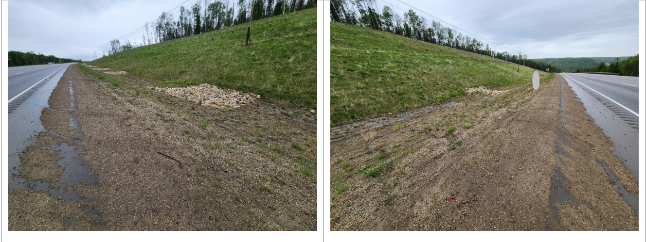
Photo 12 Pavement surface of Hwy 40:38. Note rill erosion on upper portion of slope (unvegetated gravelly material). Photos taken June 11, 2024, facing southwest and northwest, respectively.
