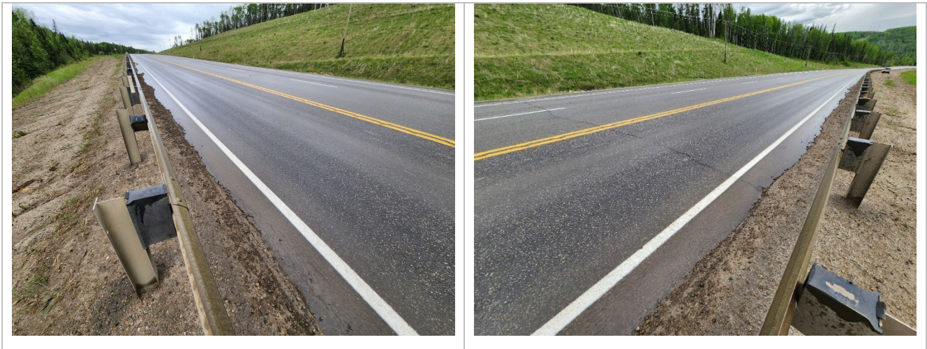
Photo 12 Pavement surface of Hwy 40:38. Note rill erosion on upper portion of slope (unvegetated gravelly material). Photos taken June 11, 2024, facing southwest and northwest, respectively.
