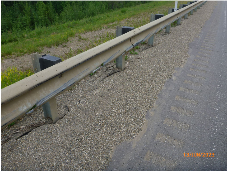
Photo 10 Section of guardrail which was struck and damaged south of site. Photo taken June 13, 2023, facing south.
