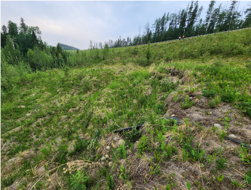
Photo 6 Exposed silt fencing near toe of slide at north/left flank. Photo taken June 13, 2023, facing southeast.
