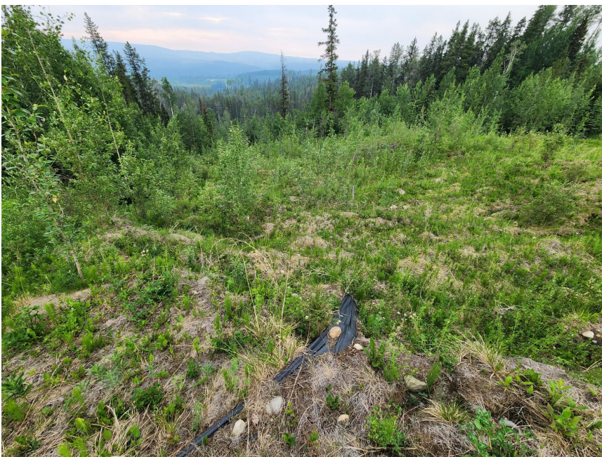
Photo 6 Exposed silt fencing near toe of slide at north/left flank. Photo taken June 13, 2023, facing southeast.
