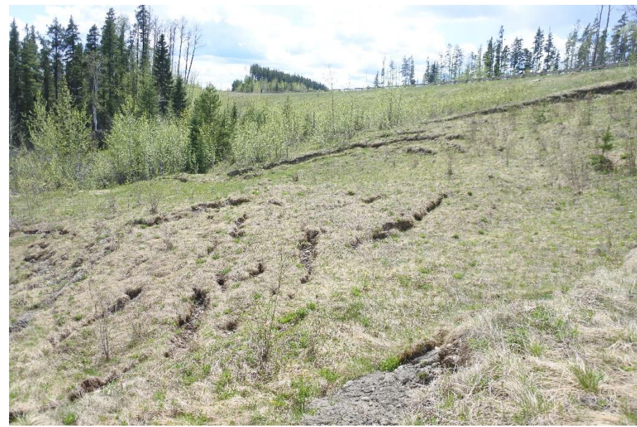
Photo 3. Looking south towards south flank of the landslide and medial tears.
