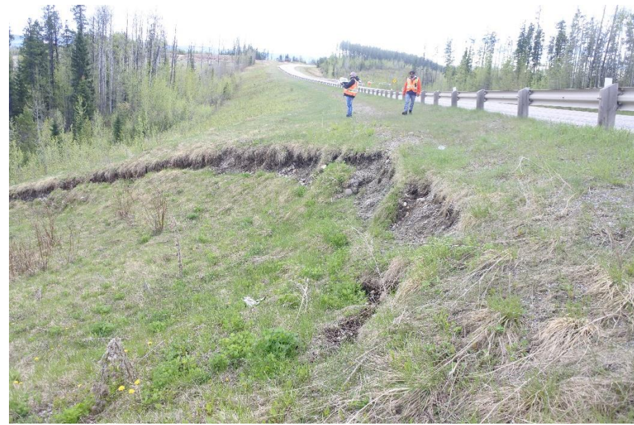
Photo 5. Looking south at backscarp which is now 2.8 m away from the highway edge.
