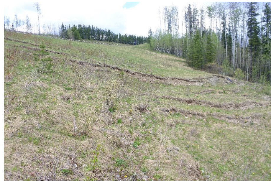
Photo 2. Looking north towards the north flank of the landslide.
