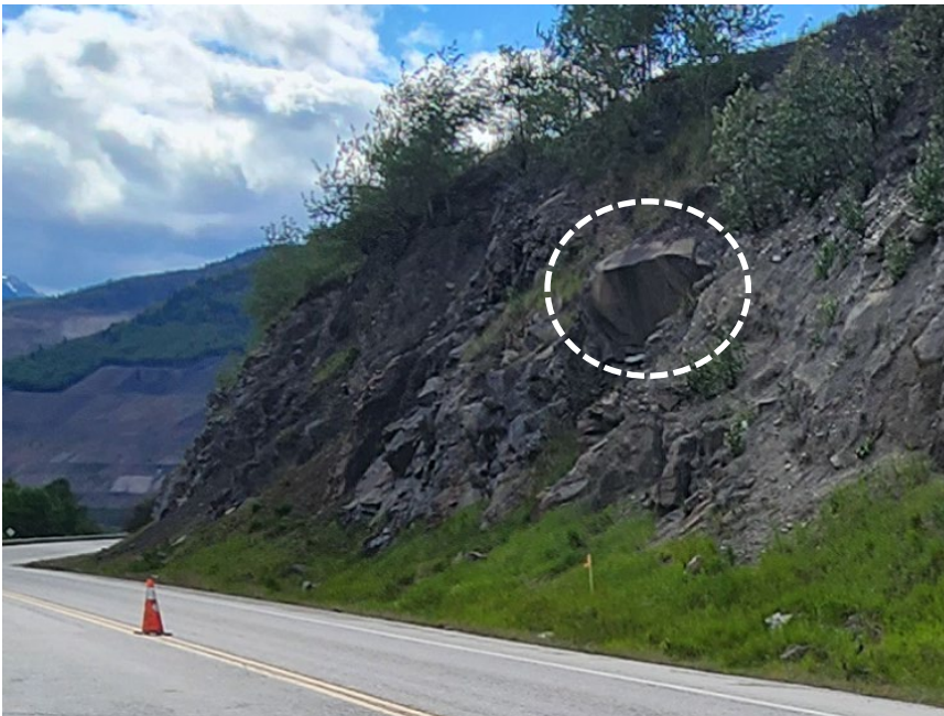
Photo 8 Large overhanging rock block (circled in white) shown in previous photo. Photo taken June 10, 2024, facing northwest.
