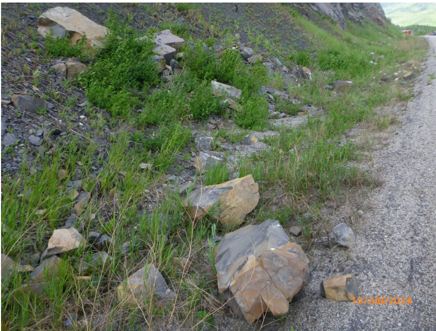
Photo 6 Rockfall particles in ditch on north side of Hwy 40:36 at GP053-II site. Photo taken June 10, 2024, facing northeast.
