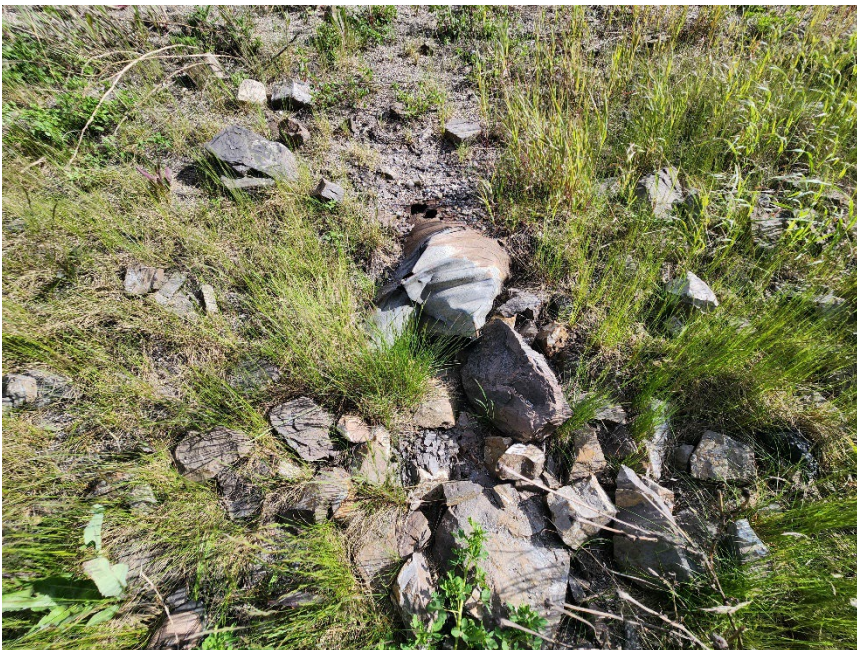
Photo 10 Culvert inlet in ditch on north side of Hwy 40:36 at GP053-I site. Culvert inlet damaged and partially blocked by rockfall particles. Photo taken June 10, 2024, facing south.
