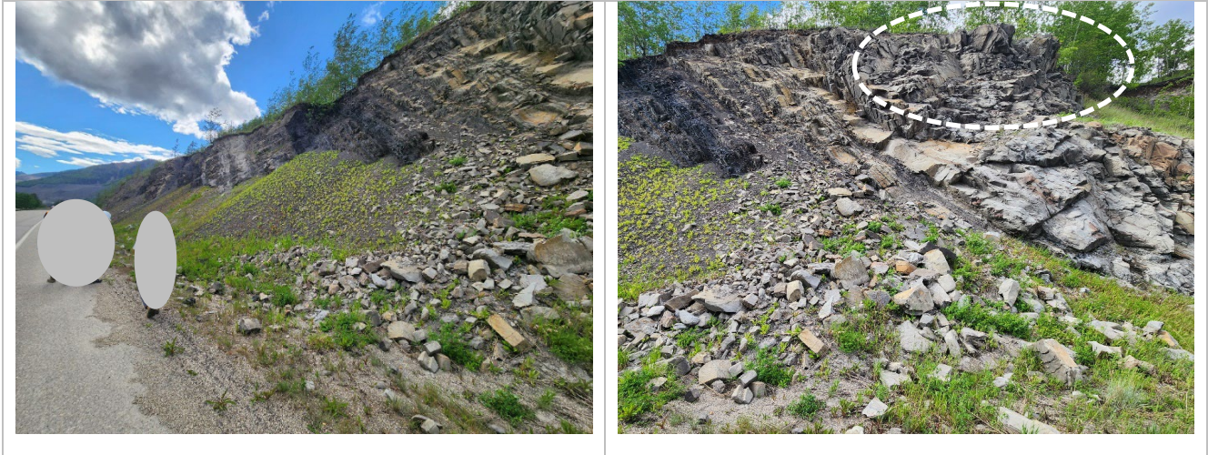
Photo 6 Rockfall particles in ditch on north side of Hwy 40:36 at GP053-II site. Photo taken June 10, 2024, facing northeast.
