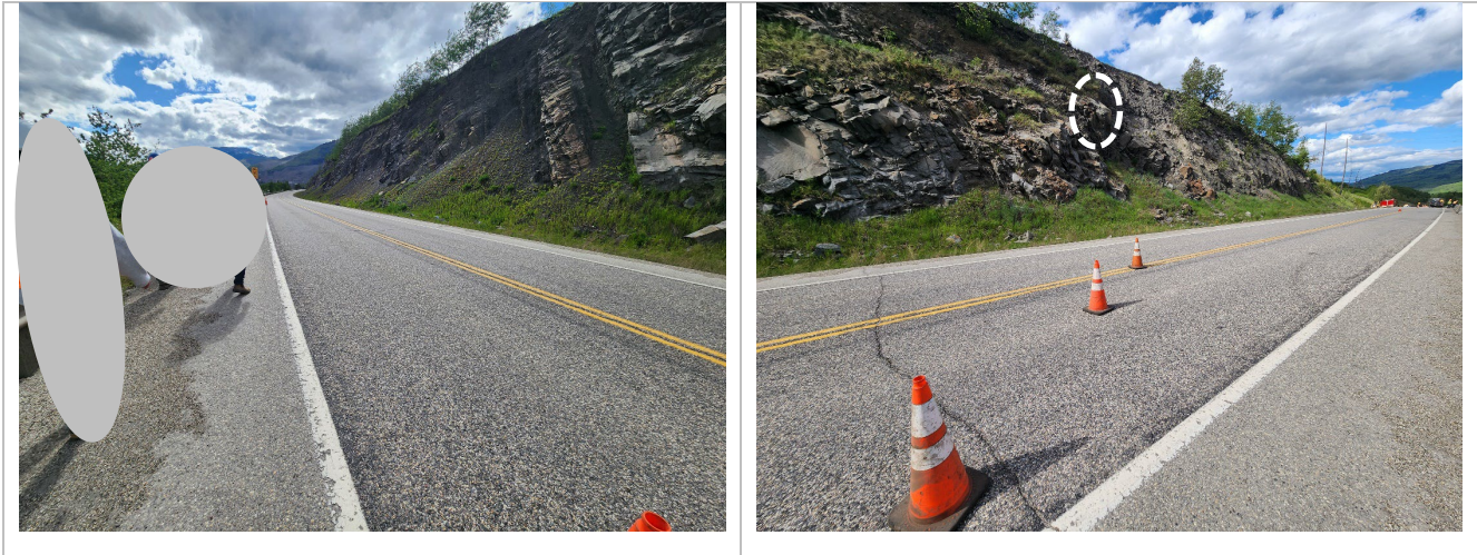
Photo 8 Large overhanging rock block (circled in white) shown in previous photo. Photo taken June 10, 2024, facing northwest.
