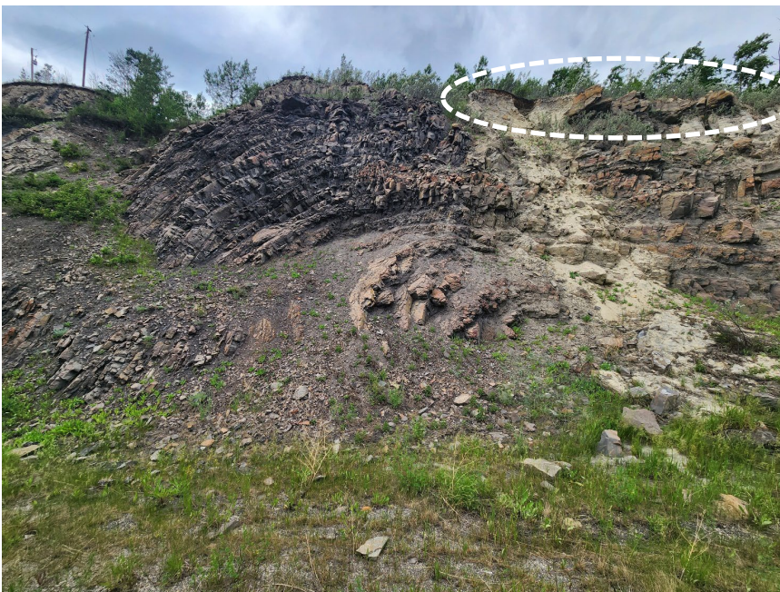
Photo 6 Fault/fold in bedrock along north side of Hwy 40:36 at GP053-I site. Note erosion and hanging rock blocks at crest of slope (some circled in white, see photo below). Photo taken June 12, 2023, facing north.
