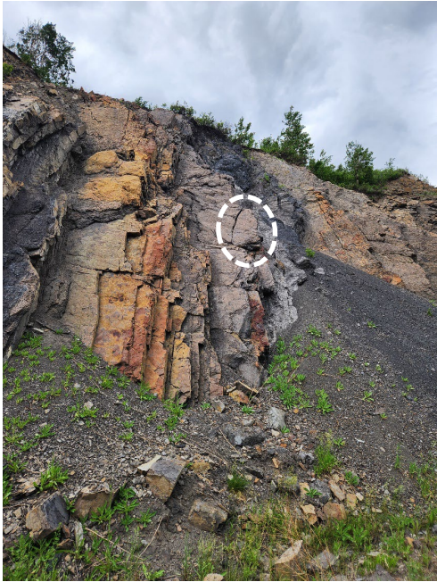
Photo 6 Fault/fold in bedrock along north side of Hwy 40:36 at GP053-I site. Note erosion and hanging rock blocks at crest of slope (some circled in white, see photo below). Photo taken June 12, 2023, facing north.
