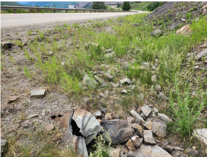
Photo 8 Crushed culvert inlet in north ditch of Hwy 40:36 at GP053-I site. Photo taken June 12, 2023, facing west.
