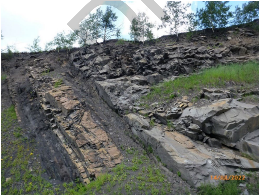
Photo GP053-II – 6 More competent, more massive layers of bedrock that are undermined do not experience as much rockfall or slope deterioration upon erosion of soft rock and coal seams. A mine access road is located behind the crest of the slope as shown in Figure 7. Photo taken July 14, 2022, facing northwest.
