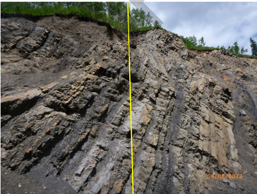
Photo GP036 – 8 Upper slope. Yellow line shows north limit of photo -6. Note uneven weathering of rock slope face which is creating overhangs and rockfall potential as well as preferential fall paths for smaller rockfall particles. Photo taken July 14, 2022, facing northwest.
