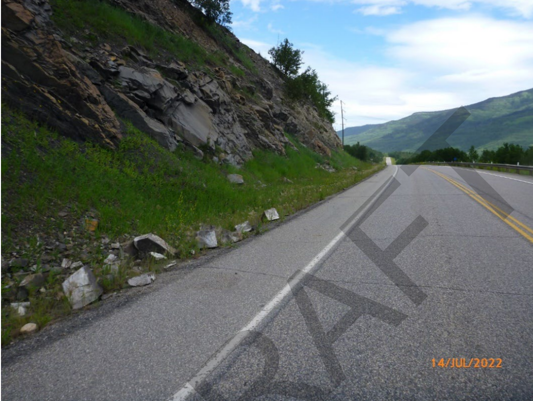
Photo GP053-II – 7 Talus slopes and rock blocks in the ditch. The rock blocks in the ditch appear to get closest to the highway by rolling down the talus slope. Photo taken July 14, 2022, facing northeast.
