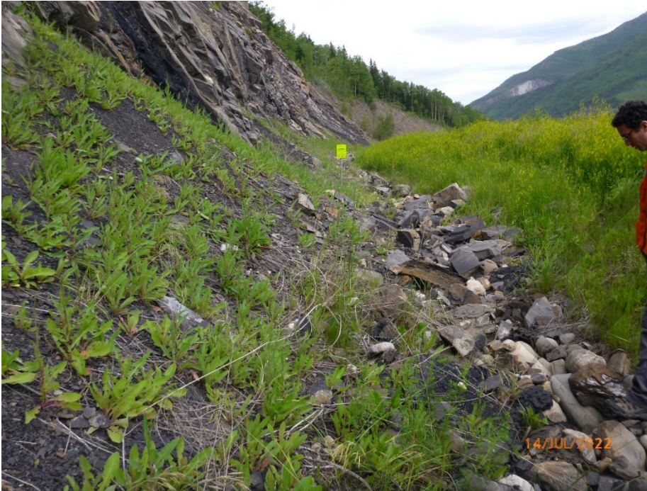
Photo GP049-II – 4 One of three observed rockfall particle 0.3 m x 0.2 m x 0.1 m located within 1.0 m from edge of pavement.
