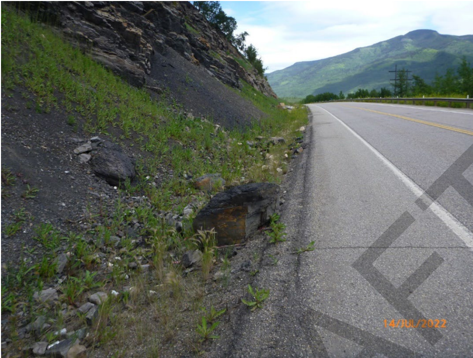
Photo GP053-II – 4 Weathered and eroded soft or highly fractured rock and coal seams are being eroded to create overhanging rock blocks which then become rock fall. Note trees at brow of slope. Photo taken July 14, 2022, facing northwest.
