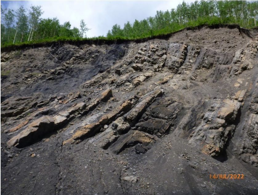
Photo GP036 – 8 Upper slope. Yellow line shows north limit of photo -6. Note uneven weathering of rock slope face which is creating overhangs and rockfall potential as well as preferential fall paths for smaller rockfall particles. Photo taken July 14, 2022, facing northwest.
