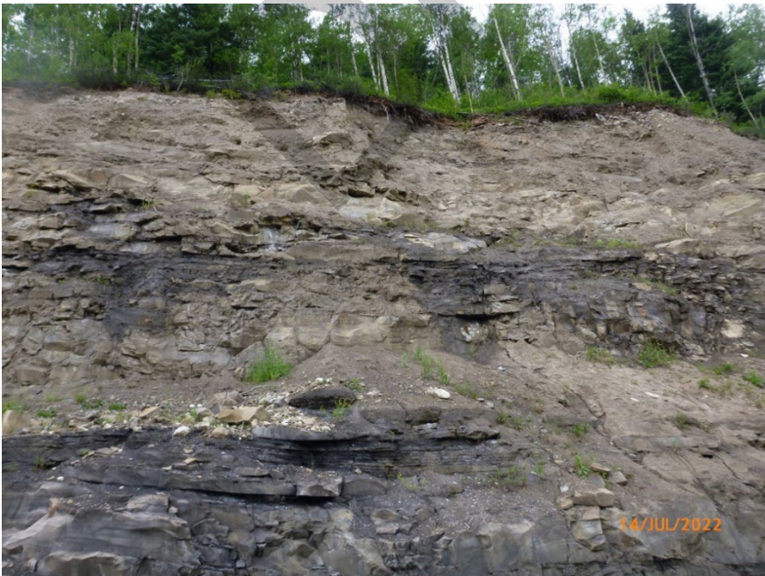
Photo GP049-I – 4 Soil at brow of slope at north end of -I site contains cobbles and rock mass looks reasonably competent. This location could be addressed with an attenuating drape. Photo taken July 14, 2022, facing west.
