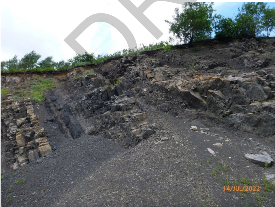
Photo GP053-II – 4 Weathered and eroded soft or highly fractured rock and coal seams are being eroded to create overhanging rock blocks which then become rock fall. Note trees at brow of slope. Photo taken July 14, 2022, facing northwest.
