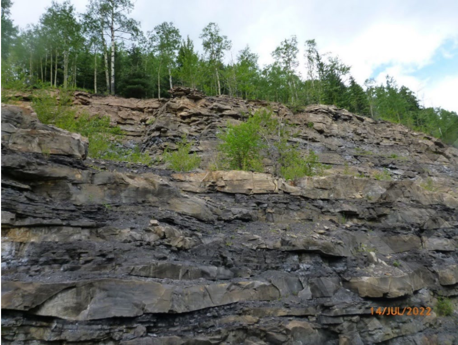
Photo GP049-I – 4 Soil at brow of slope at north end of -I site contains cobbles and rock mass looks reasonably competent. This location could be addressed with an attenuating drape. Photo taken July 14, 2022, facing west.
