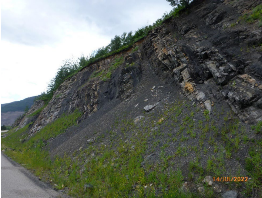
Photo GP053-II – 6 More competent, more massive layers of bedrock that are undermined do not experience as much rockfall or slope deterioration upon erosion of soft rock and coal seams. A mine access road is located behind the crest of the slope as shown in Figure 7. Photo taken July 14, 2022, facing northwest.
