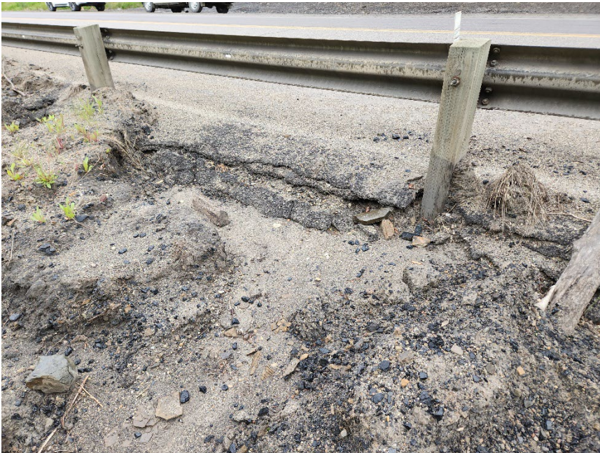
Photo 8 Subgrade exposed and edge of pavement partially undermined on east side of Hwy 40:36. Some guardrail posts also unsupported. Photo taken June 11, 2024, facing west.
