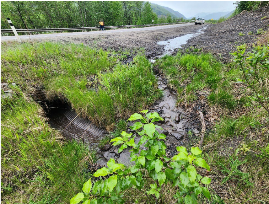
Photo 6 Inlet of culvert that conveys flow from west side to east side of Hwy 40:36. Photo taken June 11, 2024, facing south.
