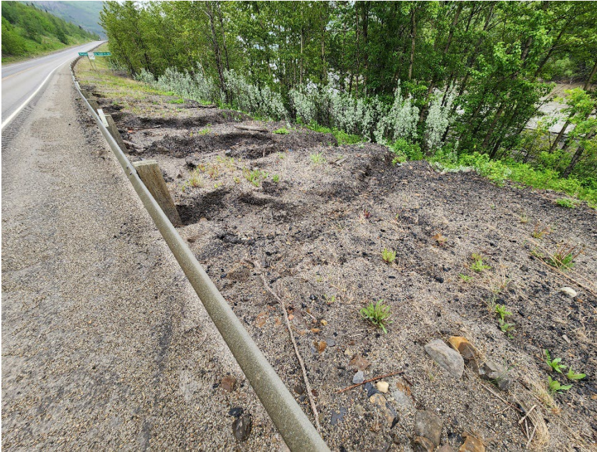
Photo 8 Subgrade exposed and edge of pavement partially undermined on east side of Hwy 40:36. Some guardrail posts also unsupported. Photo taken June 11, 2024, facing west.
