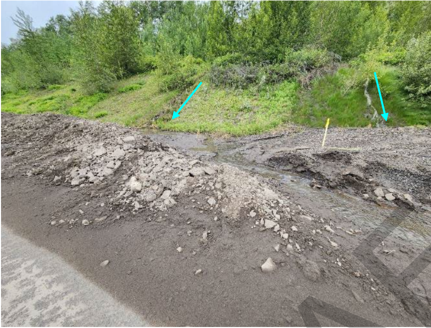
Photo 9 Temporary stockpile of debris along west side of highway between WP003 and WP009. Note survey stakes marking location of high-pressure natural-gas pipeline (indicated with red lines). Photo taken on June 22, 2023, near WP009 facing northwest.
