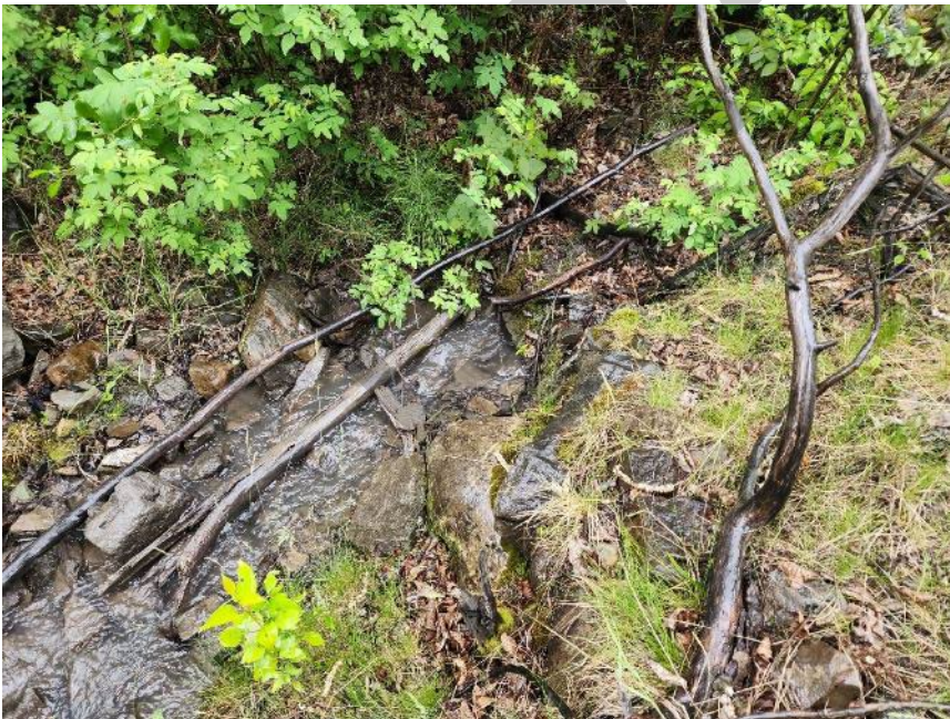
Photo 21 Flowing water exiting at downstream toe of mine slope at WP010. Photo taken June 22, 2023, facing southeast.
