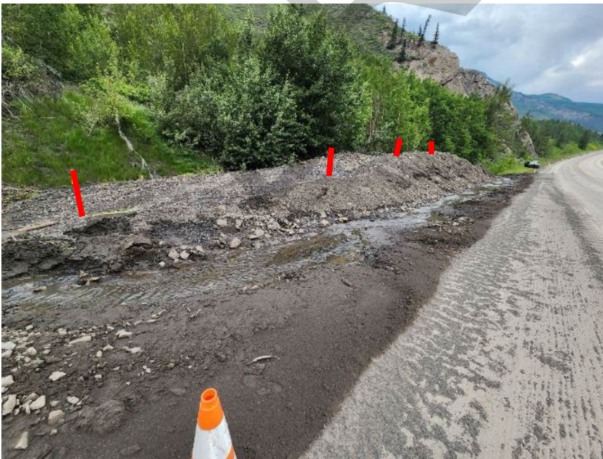
Photo 9 Temporary stockpile of debris along west side of highway between WP003 and WP009. Note survey stakes marking location of high-pressure natural-gas pipeline (indicated with red lines). Photo taken on June 22, 2023, near WP009 facing northwest.
