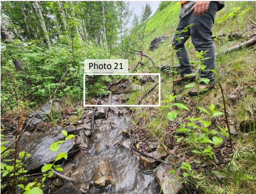
Photo 21 Flowing water exiting at downstream toe of mine slope at WP010. Photo taken June 22, 2023, facing southeast.
