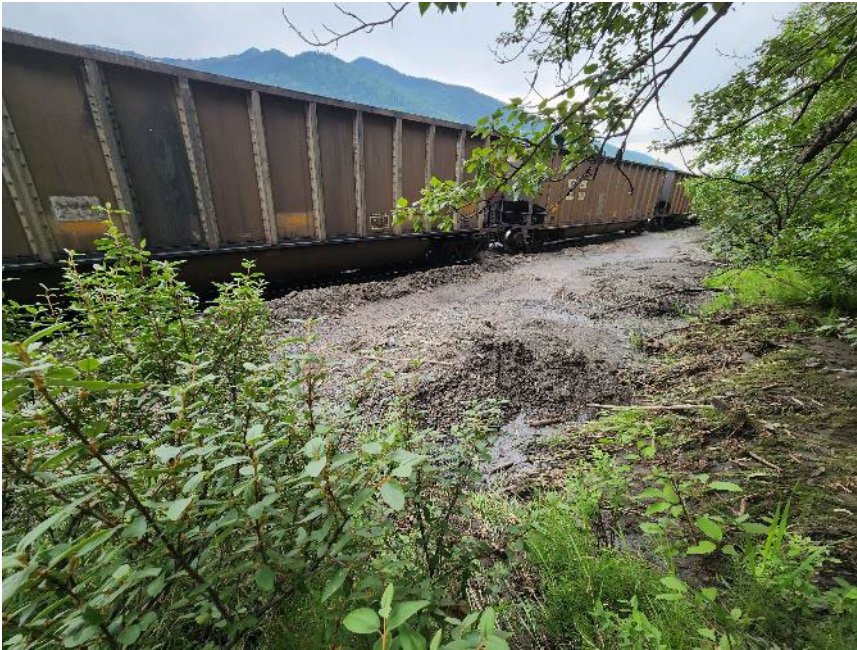
Photo 26 Debris along railway tracks. Photo taken June 22, 2023, facing southeast.
