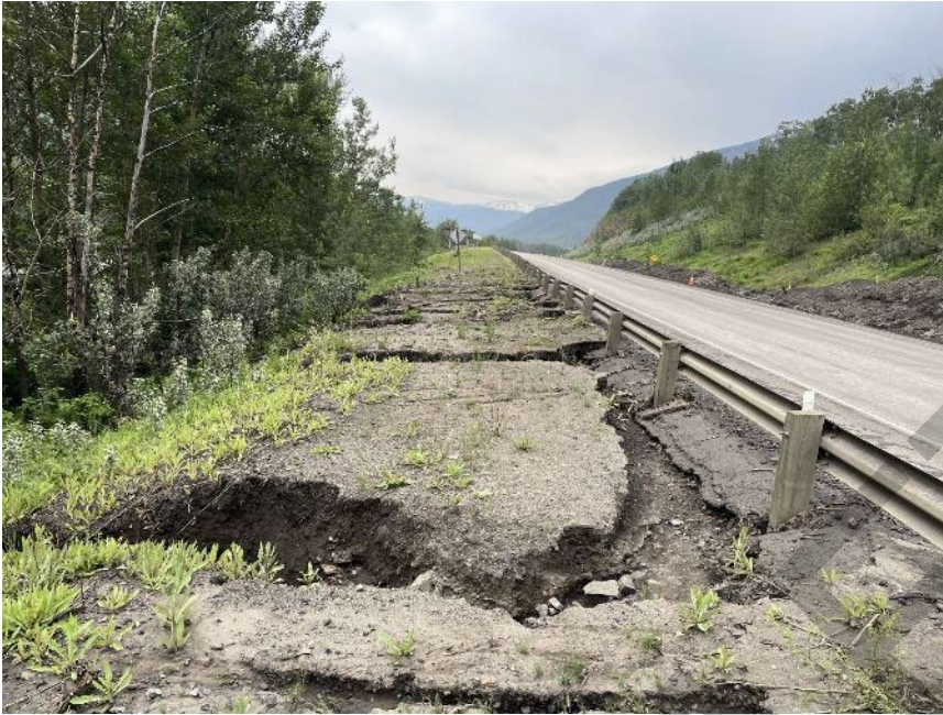
Photo 25 Pavement subgrade exposed along west side of highway, and guardrail posts partially undermined. Photo taken June 22, 2023, between WP001 and WP002 facing southwest.
