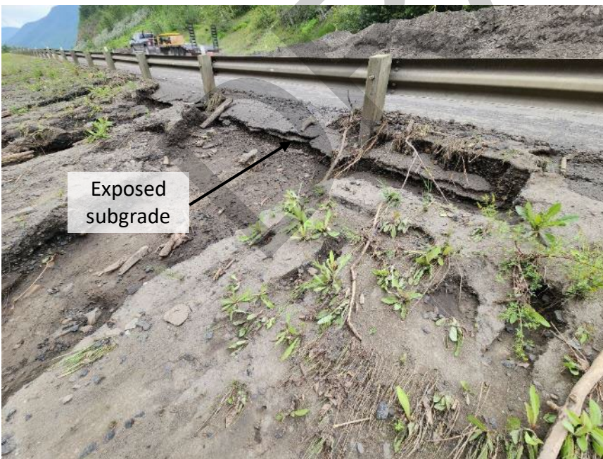
Photo 25 Pavement subgrade exposed along west side of highway, and guardrail posts partially undermined. Photo taken June 22, 2023, between WP001 and WP002 facing southwest.
