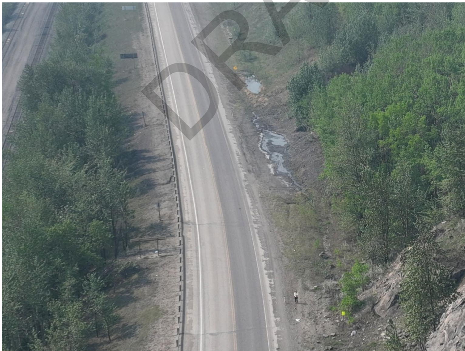
Photo 3 UAV photo of the subject debris flow site taken during our field work at the adjacent unnumbered rockfall site in May 2023. Photo taken with UAV on May 17, 2023, facing southwest.
